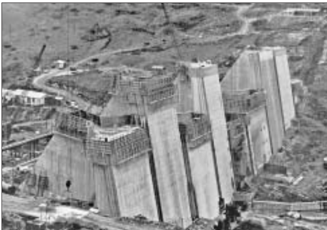
Cruachan Dam under construction [NSHEB Power from the Glens 1963, 30]
