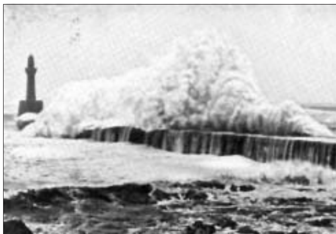
South Breakwater in a storm [postcard ca.1910]
