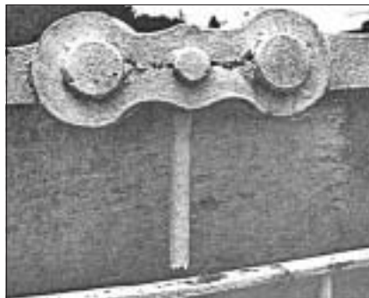
Crathie Suspension Bridge – chain detail
