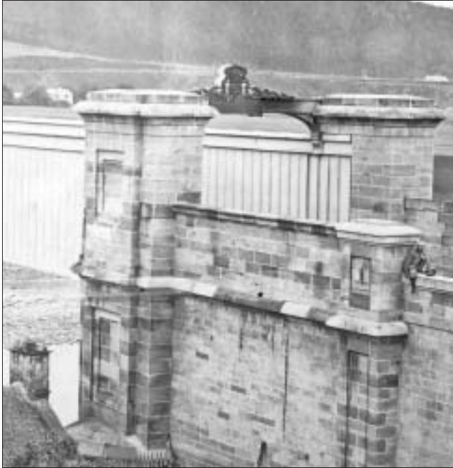
Spey Viaduct 1857 [photograph Whyte 1865]
