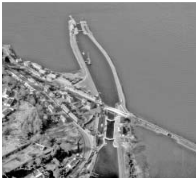
Clachnaharry Locks and Railway Swing Bridge
