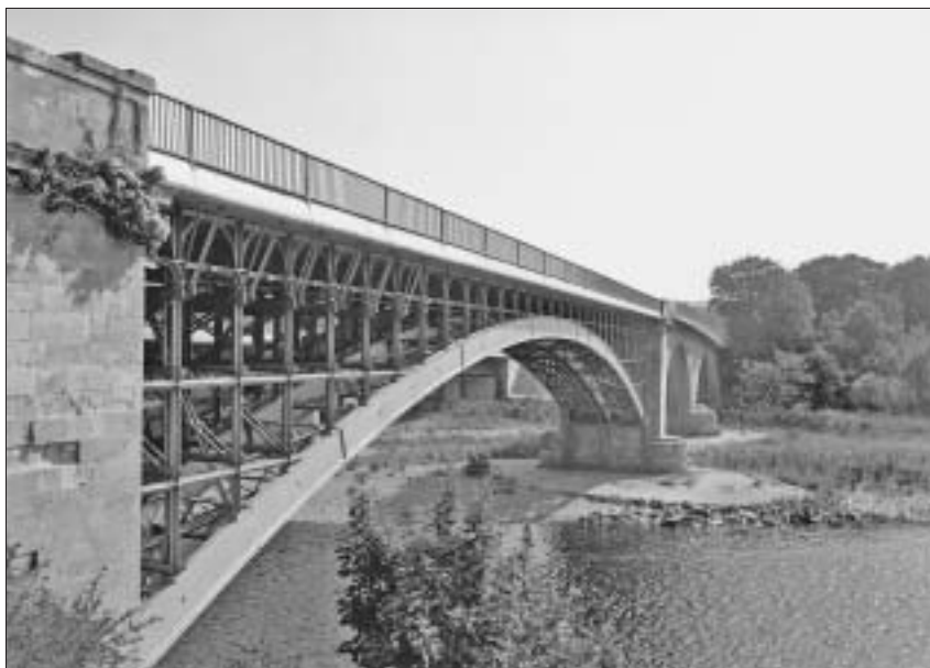
Old Spey Bridge Fochabers 1853–present
