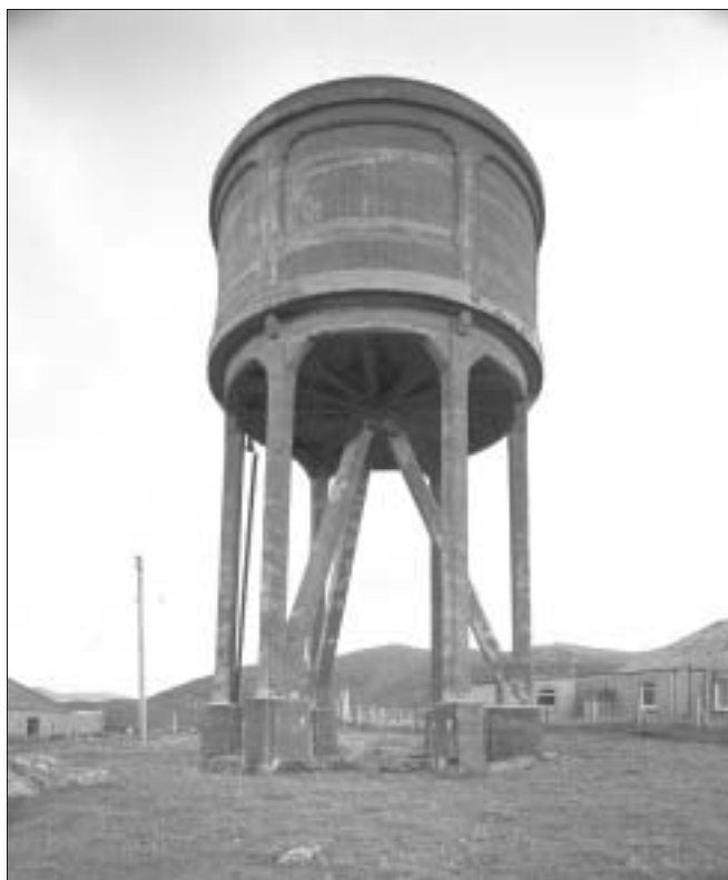
Leverburgh Water Tower
