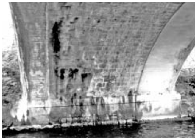
Evanton Bridge – showing original arch to Smeaton's design
