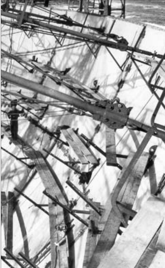
Dounreay Fast Reactor – sphere erection (lower part) [52]
