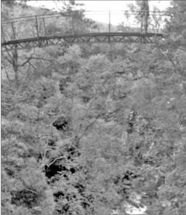
Gleann Mór Bridge
