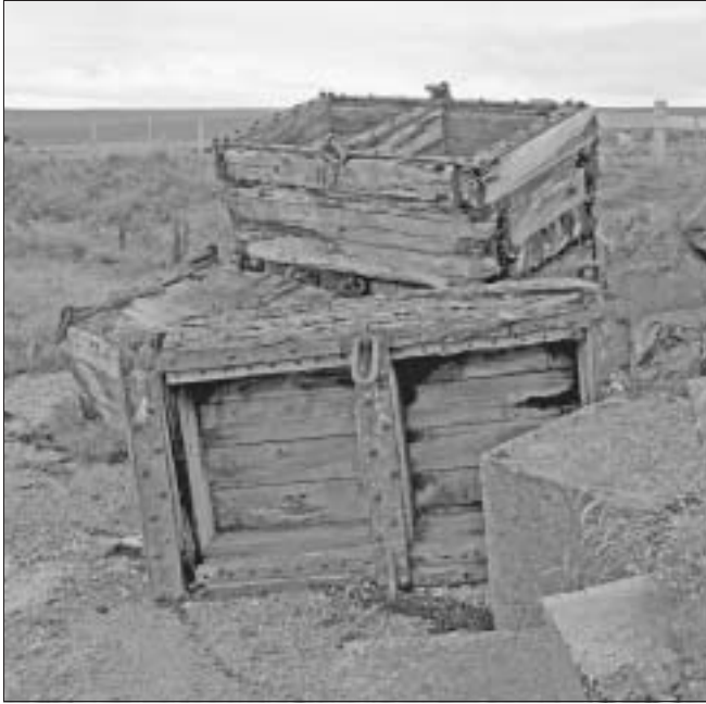
Concrete block moulds for Churchill Barrier No. 1
