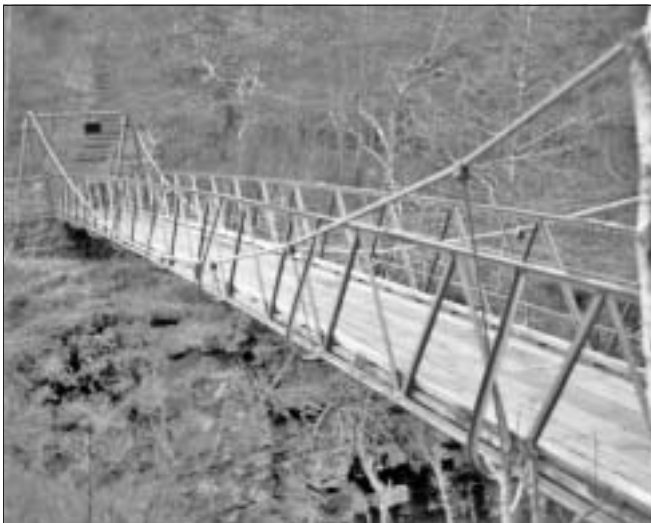
Corrieshalloch Gorge Suspension Bridge
