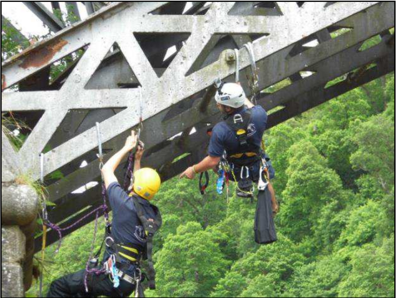
Fig. 4 Detailed inspection by Concorr in July 2014. ©Concorr
