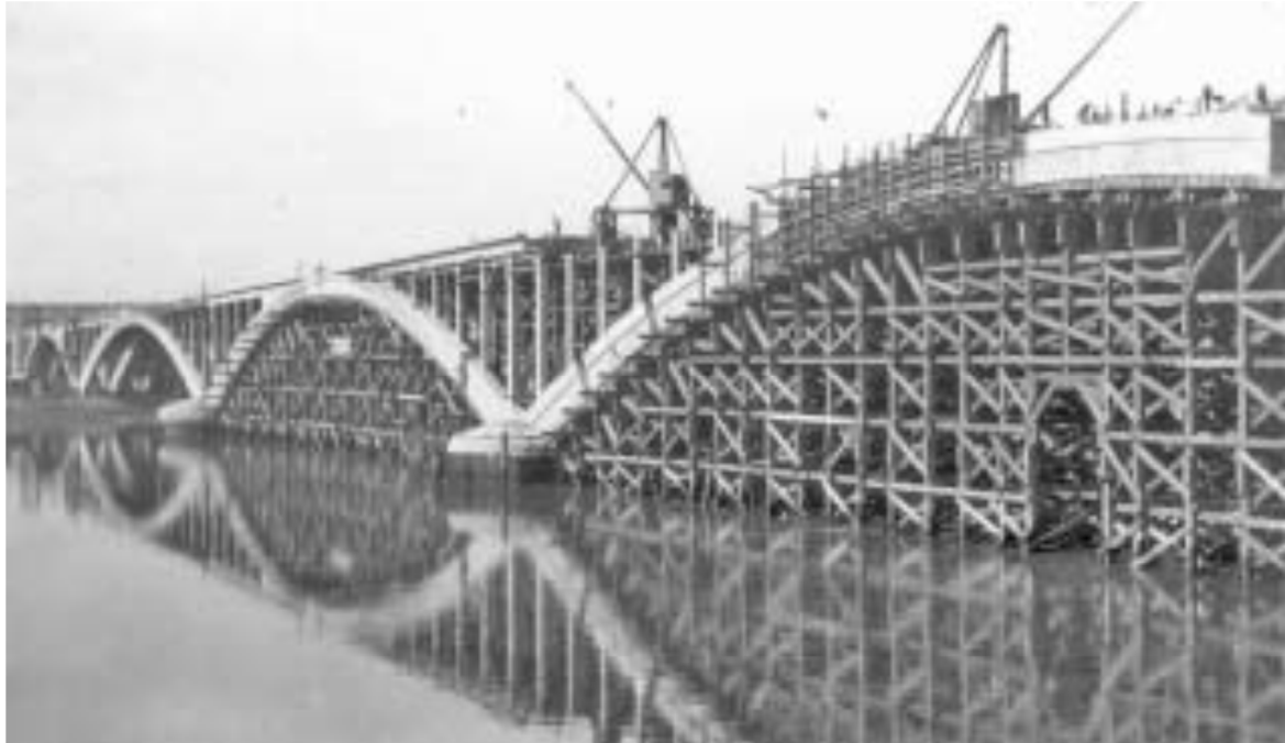
Royal Tweed Bridge under construction
