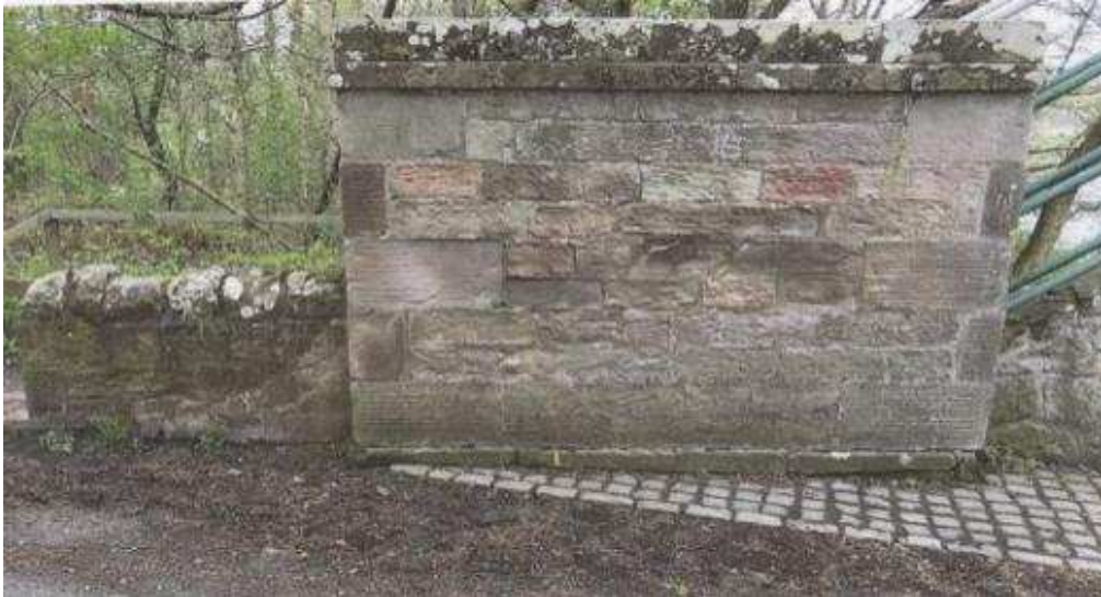
Scottish downstream 'pilaster' 1903? - note chains and cable entry at right edge [zero chainage on WARR line] ©Adrok
