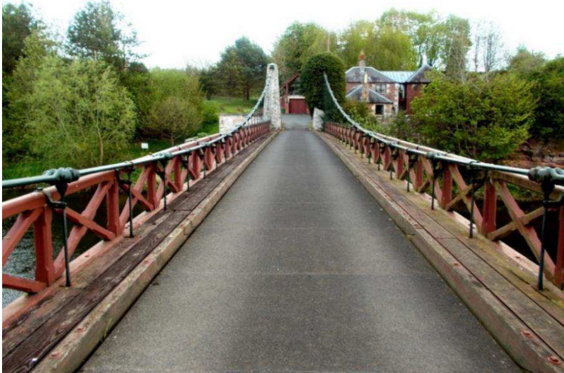
Fig. 4. Kalemouth Bridge in 2016
