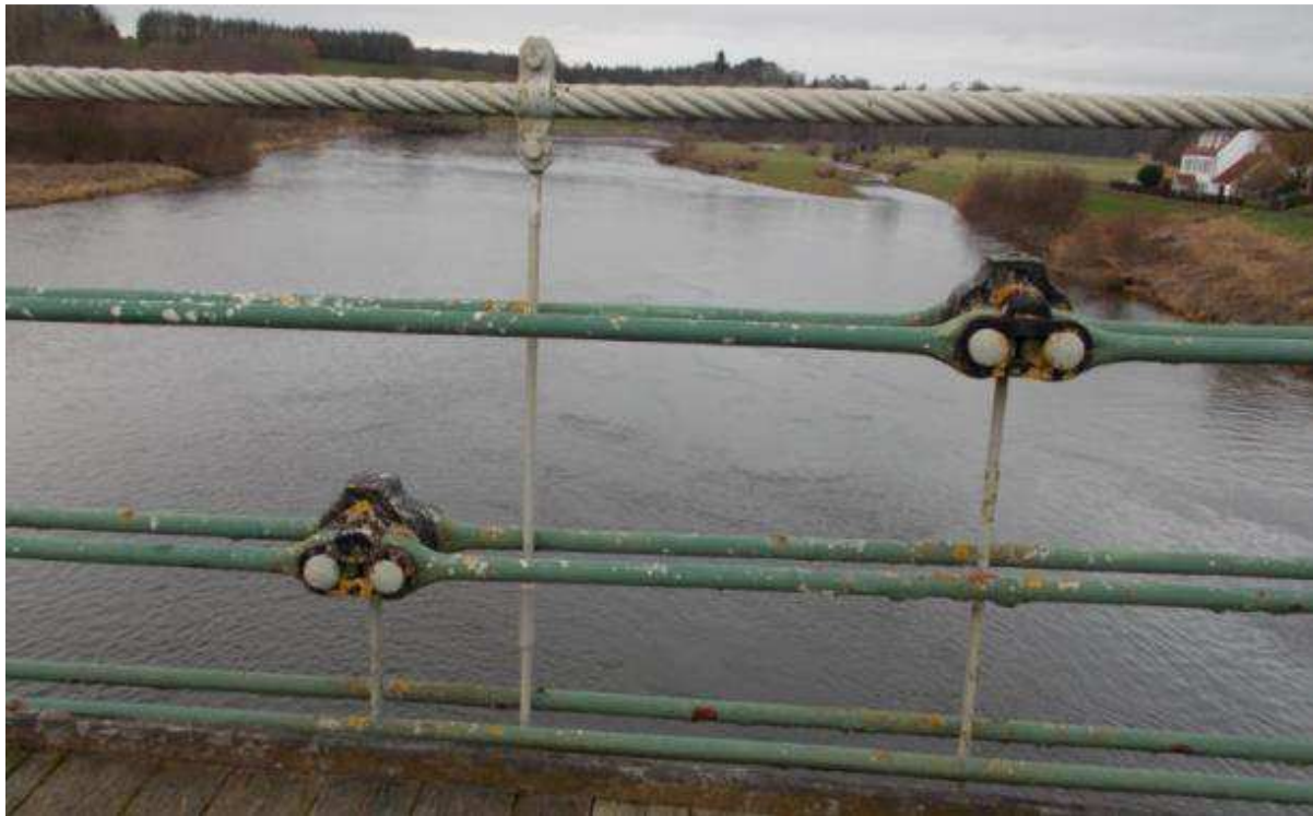
Fig. 8. Union Bridge’s 1820 chains with 1903 strengthening cable
