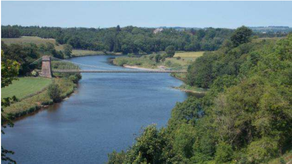
Fig. 9. Union Bridge in 2015
