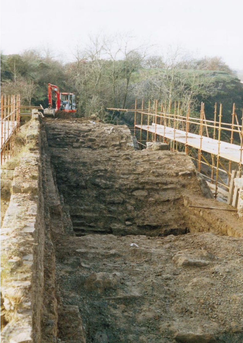
Fig. 12. South span-drel wall and undressed extrados of arches
