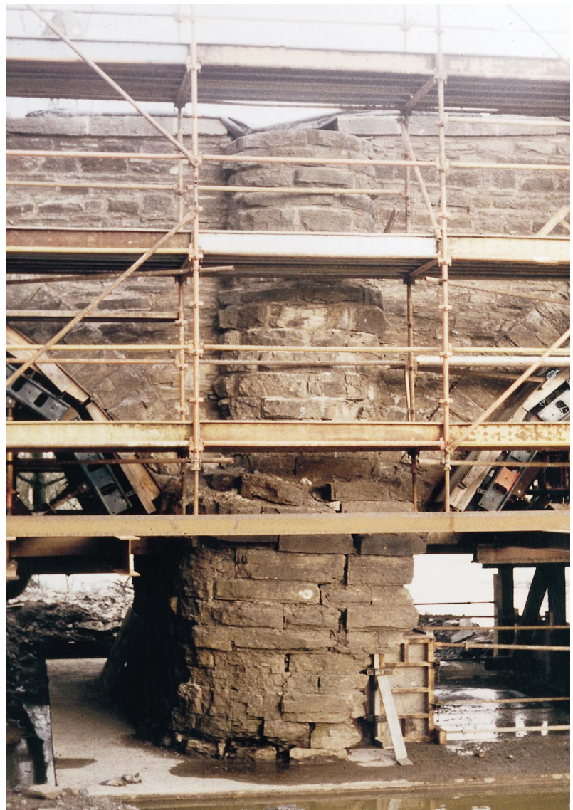
Fig. 18 (below). West pier, west side—pointing and concrete surround to base
