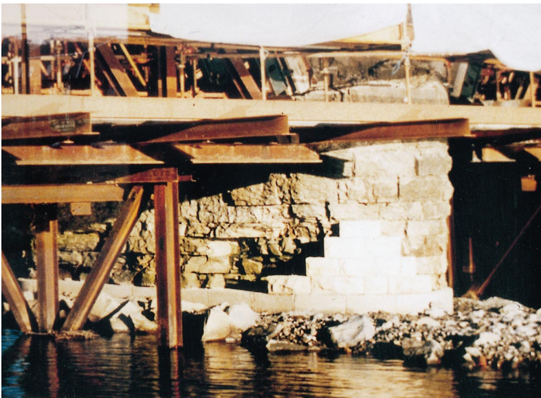
Fig. 19 (top). Non-structural concrete spandrel infill before waterproofing
