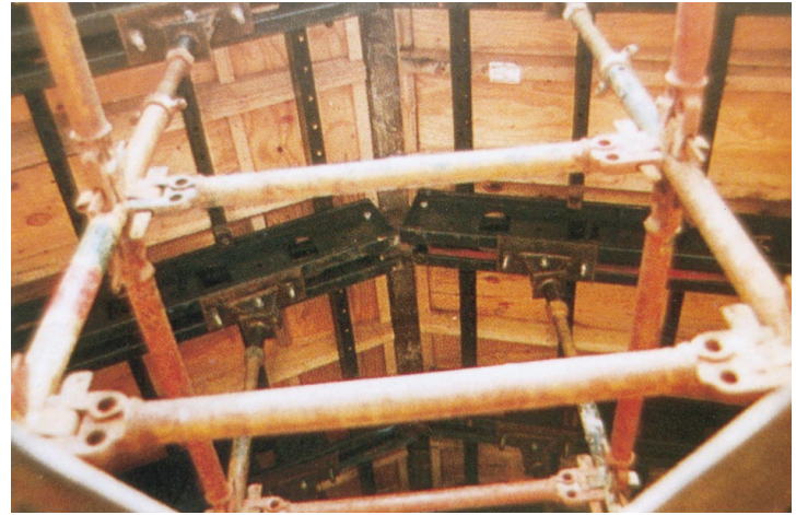
Fig. 16 (above left). Skate used for sliding temporary support frameworks into place
