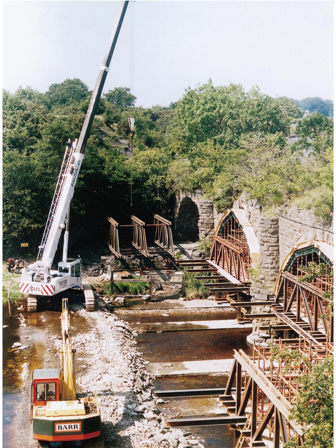
Fig. 15. State of work on 3 August 1995 with water lowered at viaduct
