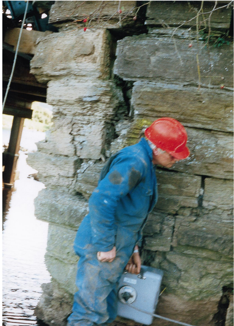
Fig. 13. West pier — radar scanning with Oyo receiver
