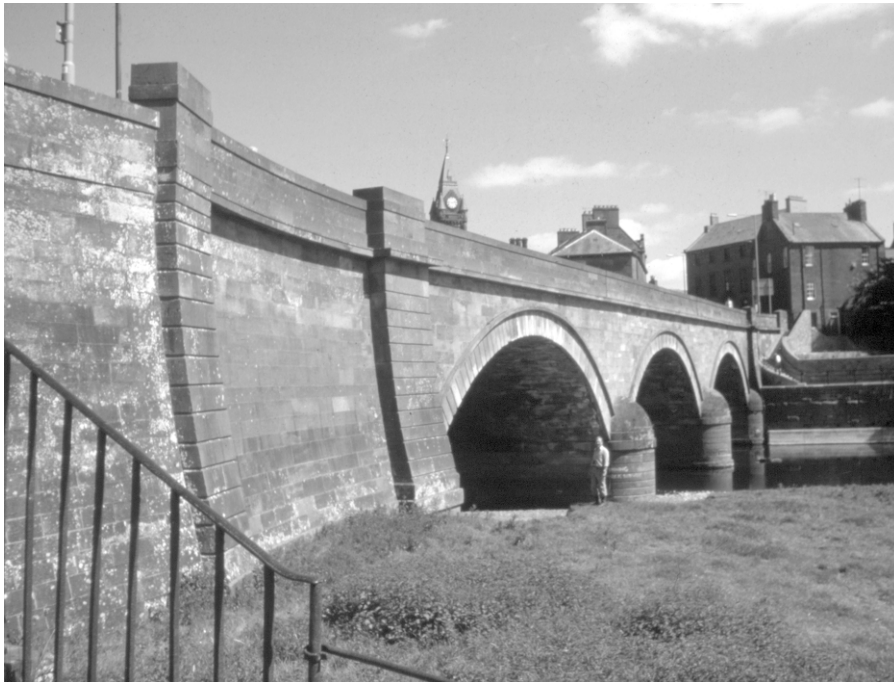
Annan Bridge, Dumfriesshire
