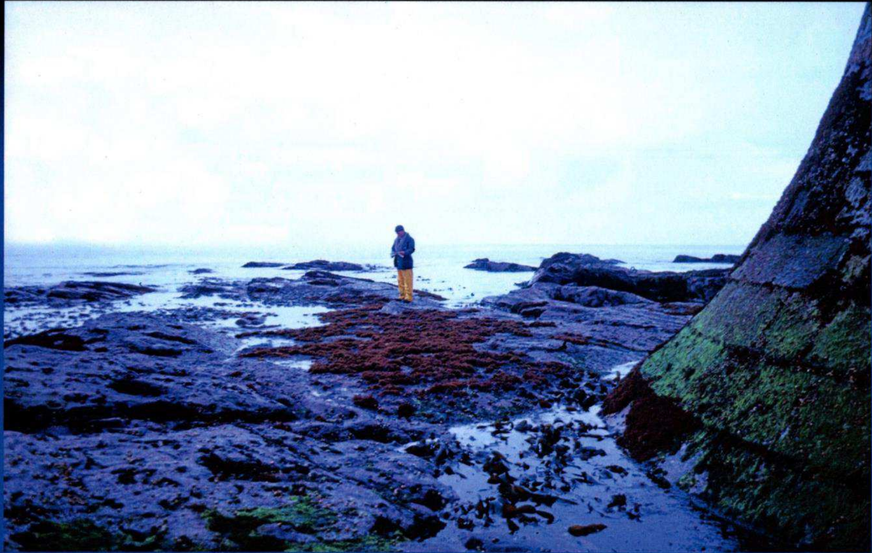
The base of the lighthouse as inspected by the writer in 1986
