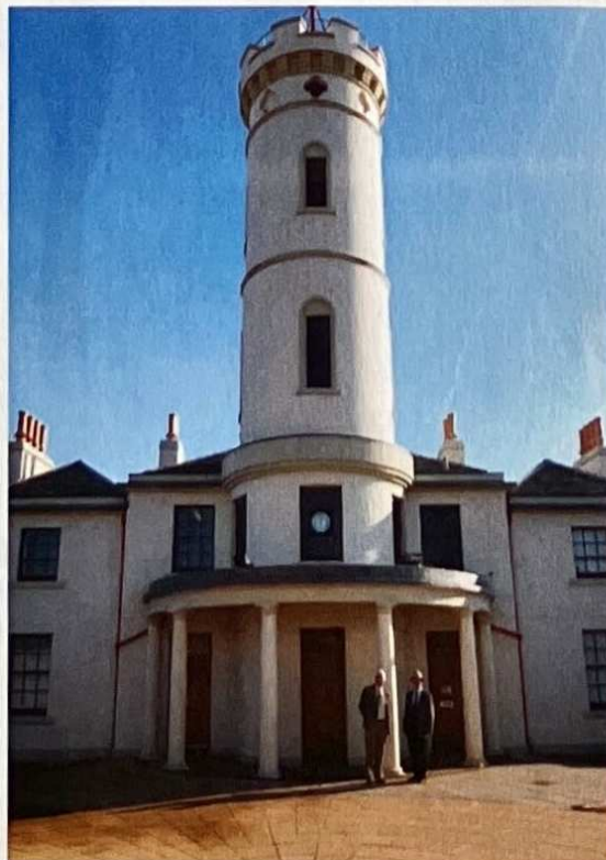
The Signal Tower Museum, Arbroath. Completed in 1813 as the Bell Rock Lighthouse Shore Station
