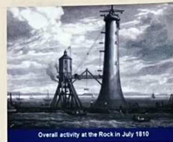
Fig.8 Progress of work nearing completion
