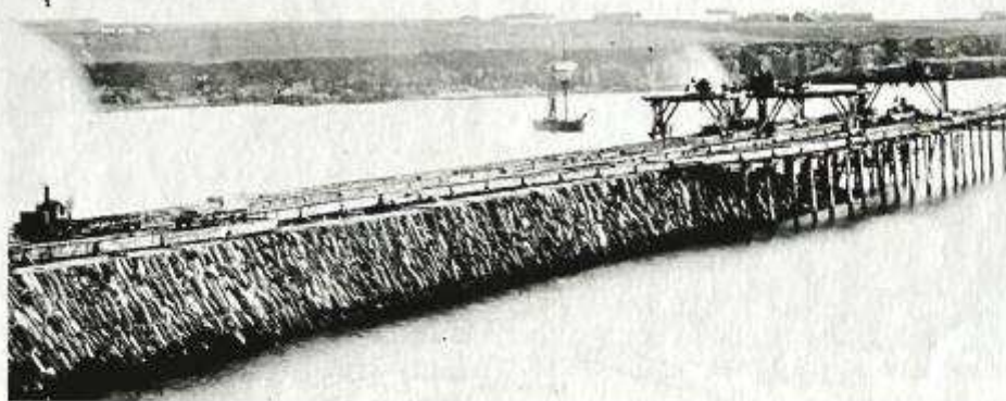
Fig. 19 Wick Breakwater 1868 – railway and travelling frames © Wick Society
