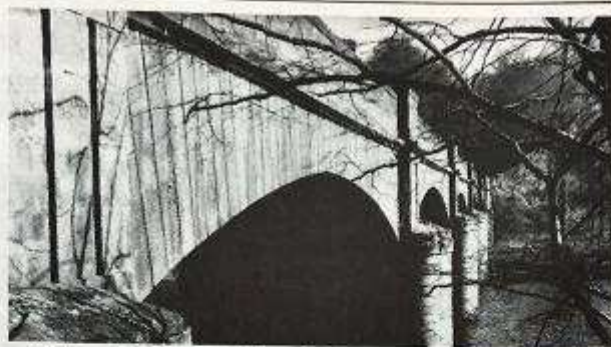
Mertoun Bridge was designed by James Slight of Edinburgh and was originally built with wooden arches between the stone piers and abutments. The graceful stone arches seen in this photograph were added later.
