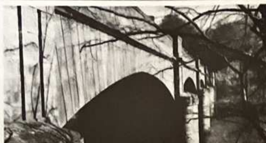
Mertoun Bridge was designed by James Slight of Edinburgh and was originally built with wooden arches between the stone piers and abutments. The graceful stone arches seen in this photograph were added later.
