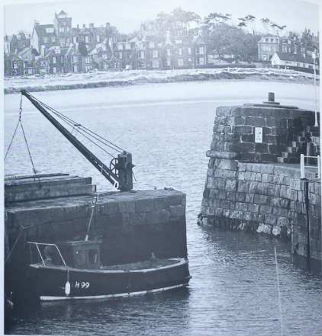
[23] North Berwick Harbour, improved c. 1812. Robert's specification for rebuilding the destroyed north pier (on right) is dated 5 Aug. 1812. The extent to which it was implemented is uncertain.
