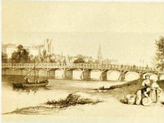
[30] Temporary bridge over r. Clyde at Portland Street, Glasgow, 1832-46.
