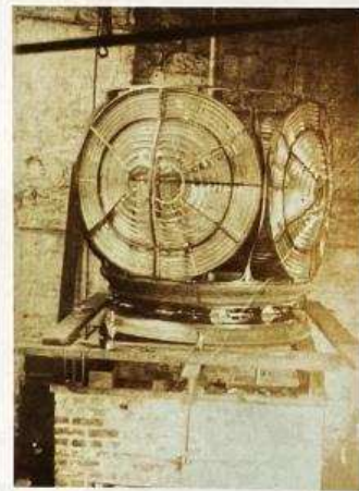
[118] Charles's equiangular spherical prism refractor for Fair Isle Lighthouse c. 1890.
