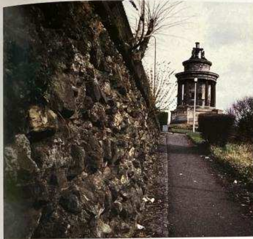
[34] Regent Road retaining wall c. 1818 and Burns' Monument, 1830.
