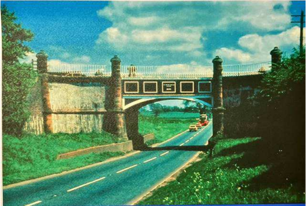
Birmingham & Liverpool Junction – Stretton Aqueduct
