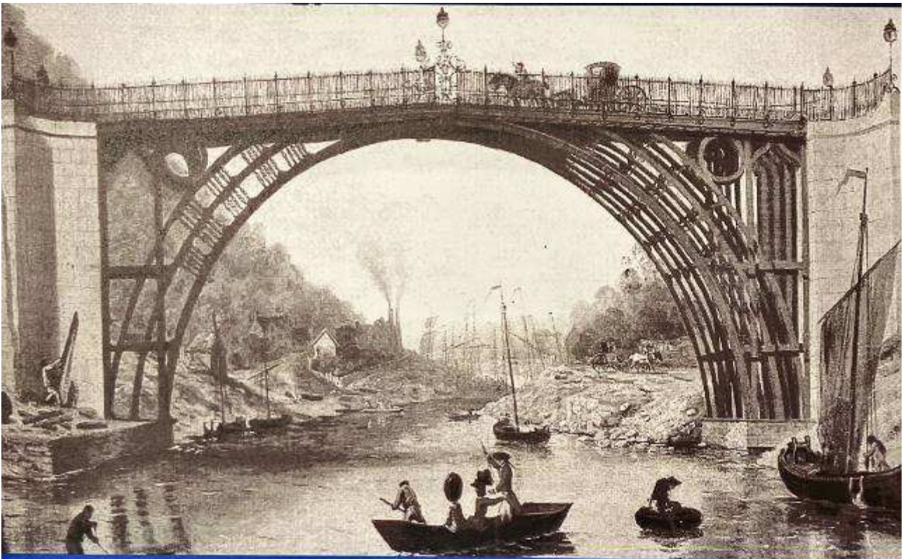
The Iron Bridge, Coalbrookdale 1779 – 80 Span 100½ ft 380 ton Designer: A. Darby III influenced by T. F. Pritchard architect (Blackfriars Br., London 1769 had a 100 ft central stone span)
