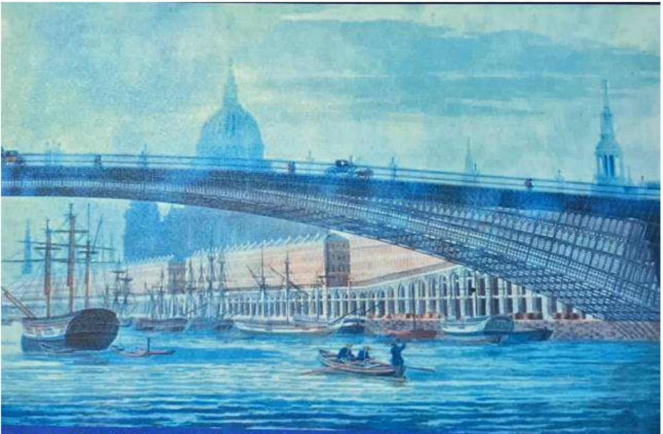
London Bridge – Telford's proposed 600 ft cast iron span 1800-01, still under consideration until the 1820s
