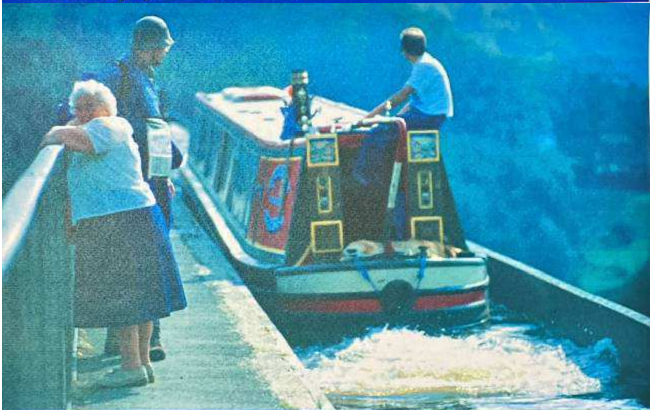
Pontcysyllte Aqueduct, Ellesmere Canal 1795-1805 'Supreme structural achievement of the Canal Age'
