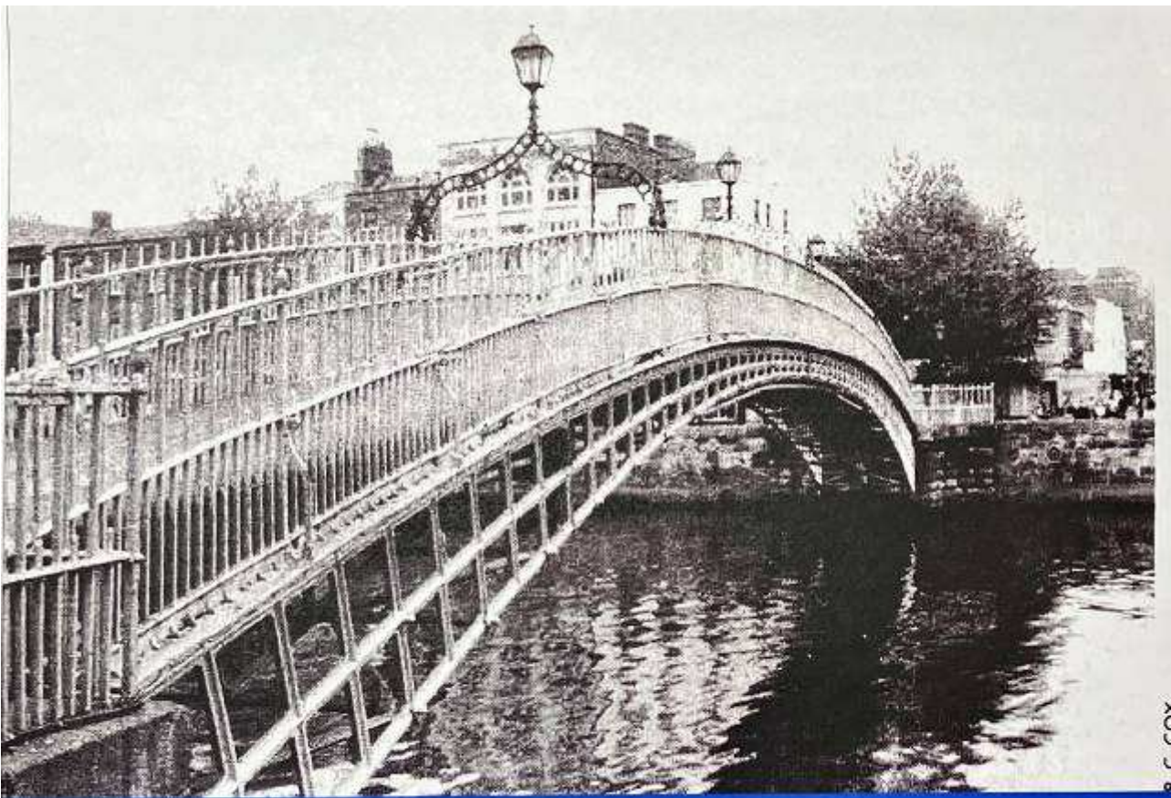
Liffey ft/br 137 \frac{3}{4} ft span influenced by Telford's smaller iron bridges
