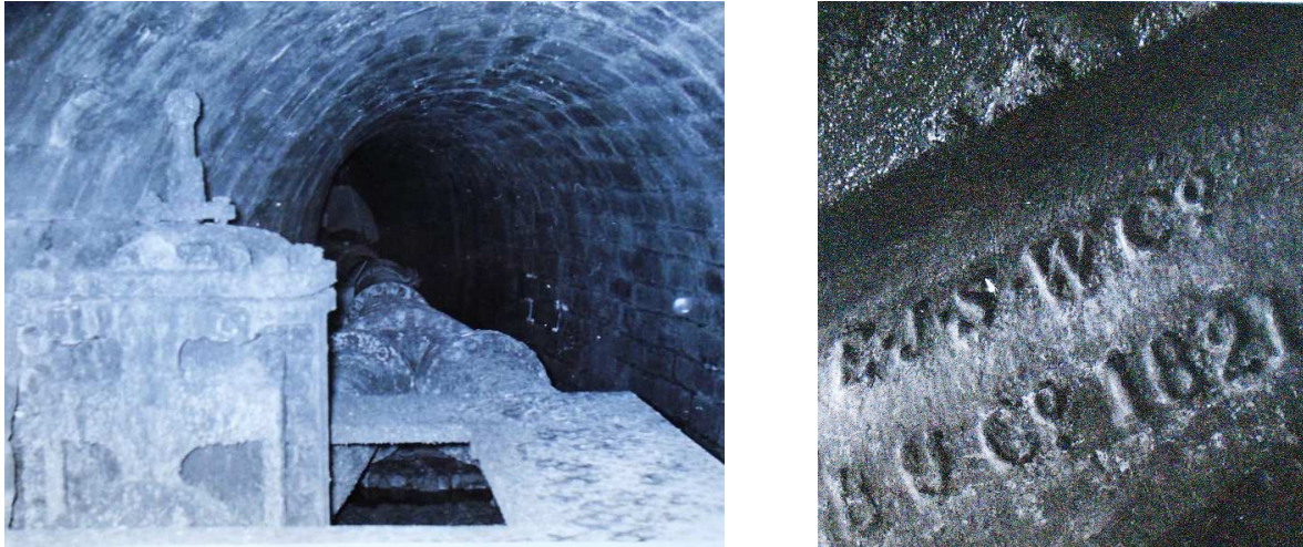
Fig. 12. Butterley Co. 18in dia. Crawley to Hanover St iron main in Castle Hill laid 1822 + reservoir branch
