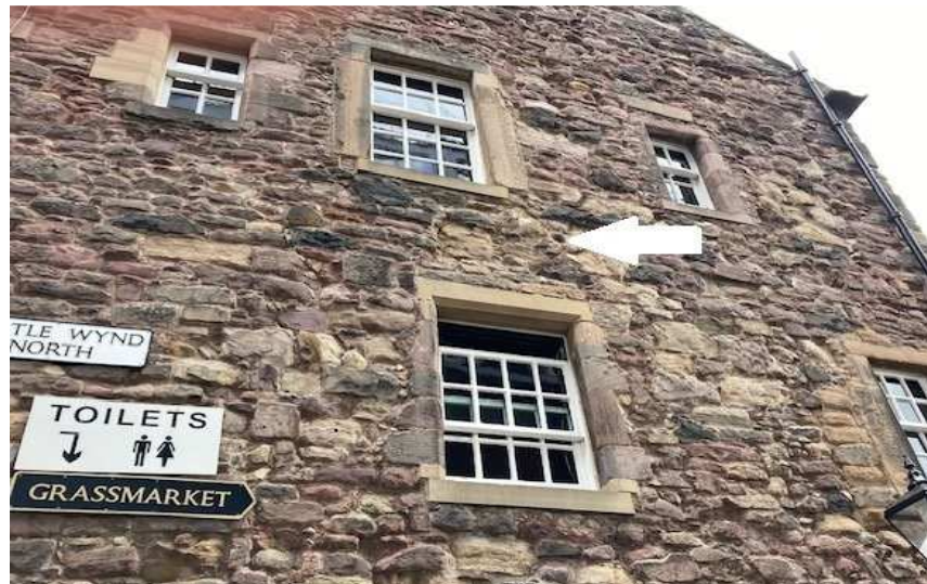
Fig. 6. Cannon-ball at Cannon-ball House, Castle Wynd, opposite Weaving Mill showing water level at Comiston Cistern 14,637ft (4.5km) south [Scots Mag 1760]
