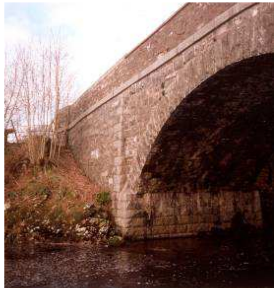
Cay's Glenlair road bridge – 45ft span © K..McCrae
