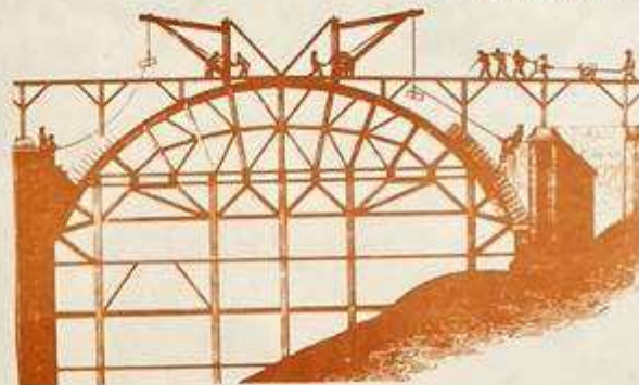
Dean Bridge. Forming arches. Note machinery, scaffolding and modus operandi .
