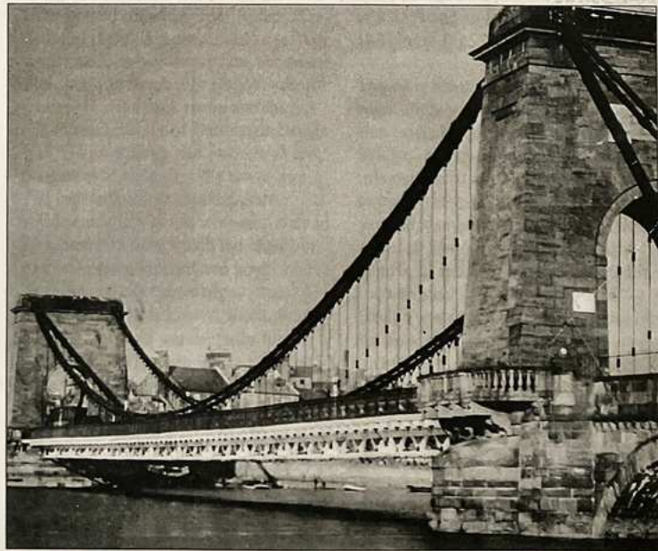
Fig. 12. Montrose Bridge 1829-1927, timber trussing showing below the deck (Davidson postcard)
