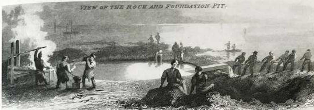
Forging beacon fixings and pumping foundation pit, June 1808 (3, pl. XI)
