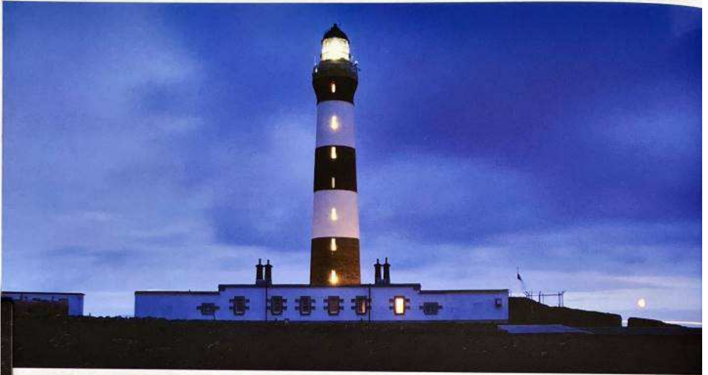
Above: North Ronaldsay Lighthouse, Orkney, designed and built by Alan Stevenson. Established 1854. This light replaced the original beacon established by Thomas Smith in 1789.
