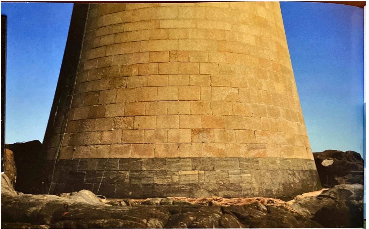
Above: Skerryvore Lighthouse – base of tower (see page 12)
