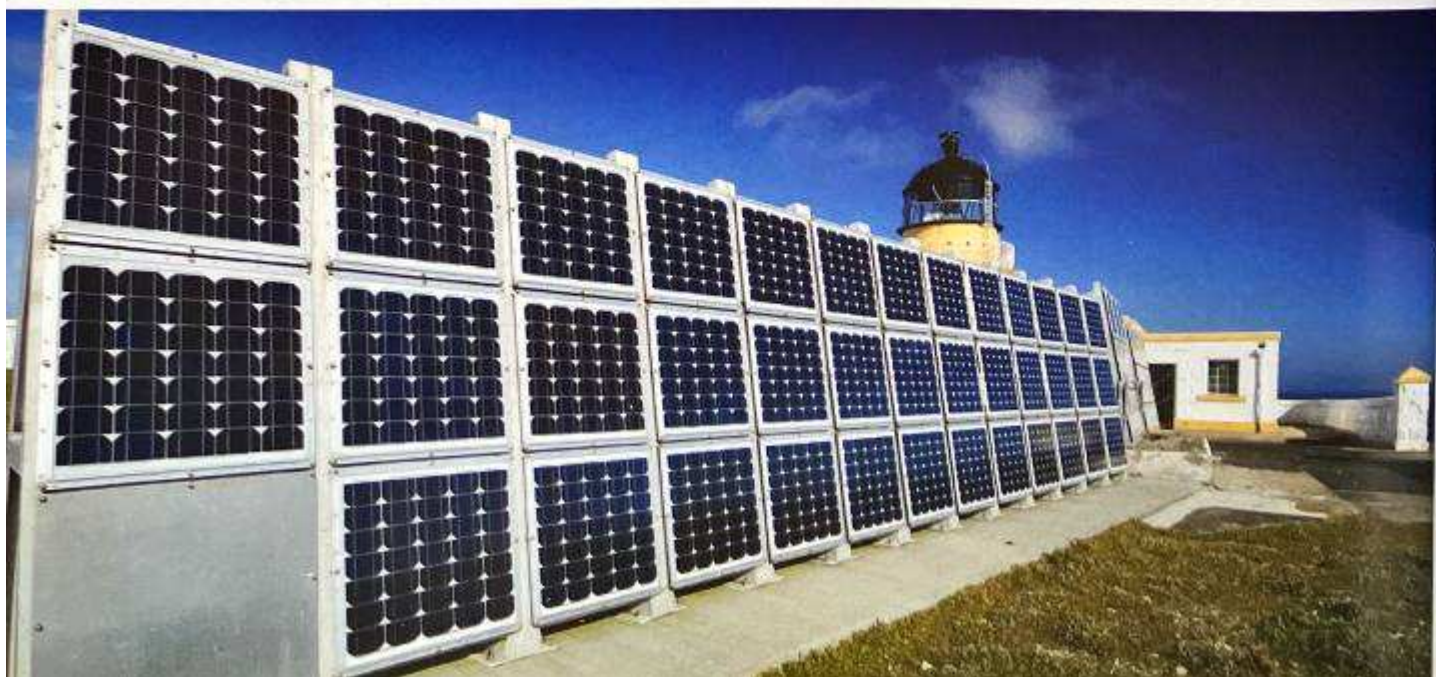
Below: Fair Isle North (Skroo) built by David A. Stevenson. Established 1892. The solar panels were added in 2006.
