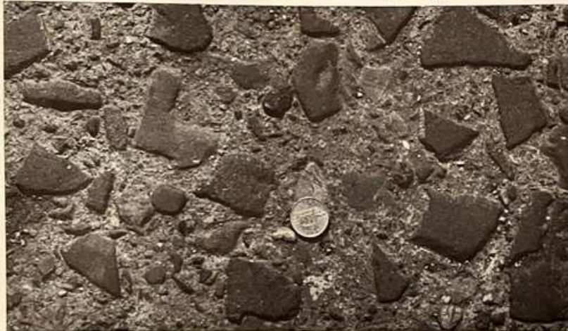
Figure 6. Close up of the concrete surface at High School Yards.
