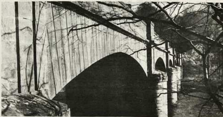
Fig. 13 (top left). Dean Bridge under construction in 1831 from Telford Atlas 1838
