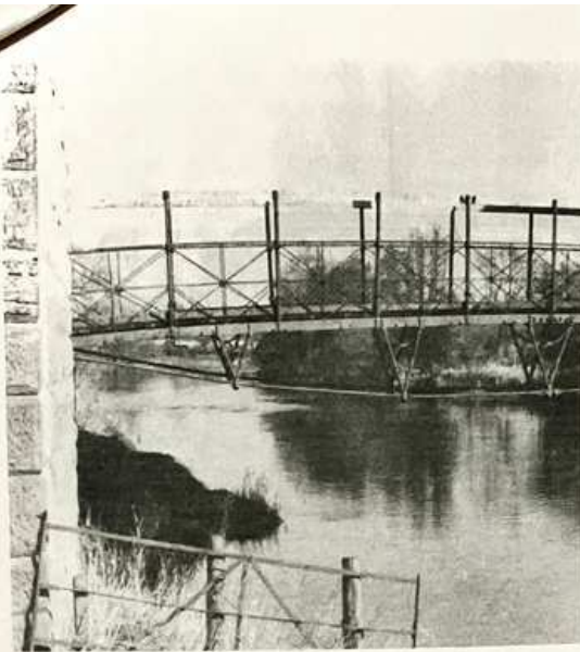
Fig. 35. Roxburgh Viaduct Footbridge (NT 702304)
