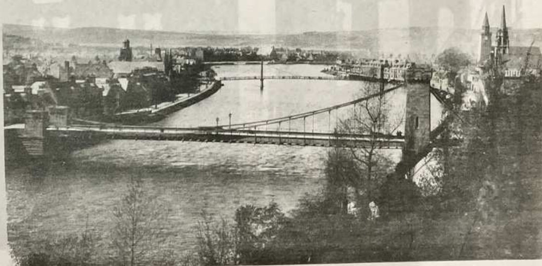
Fig. 34. Inverness Suspension Bridge, August 1983
