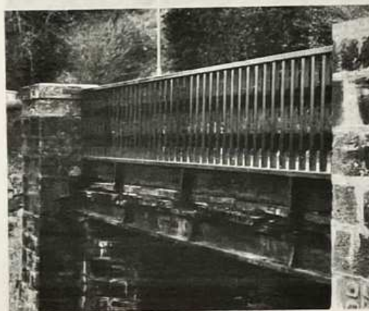
Fig. 20 (left). Clachnaharry Bridge on A9, Inverness (NH 645465); girders cast by the Falcon Foundry, Inverness
