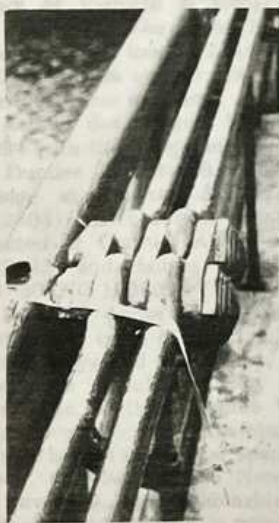
Fig. 29. (Above) Union Bridge — interconnecting link and hanger saddle detail (cross-pins do not connect the two main chains); (left) Kalemouth Bridge — cross-pins connect the main chains
