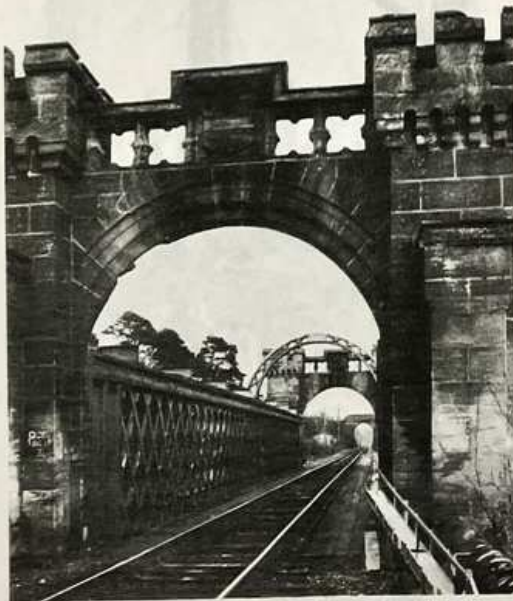
Fig. 37. Tilt Viaduct, Blair Atholl (NN 874652)
