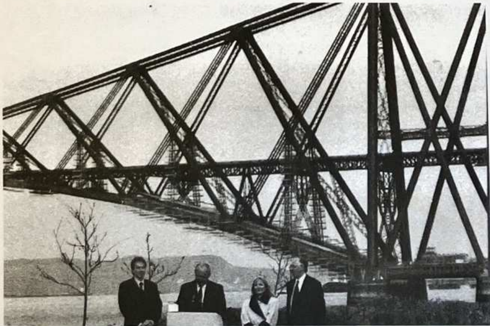
Figure 11 – Bridge Maintenance at the Time of Mr. Tony Blair P.M's Visit
