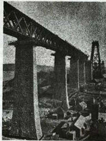
Figure 8. Completing a central girder. Vernon-Harcourt (1902). Civil Engineering .
