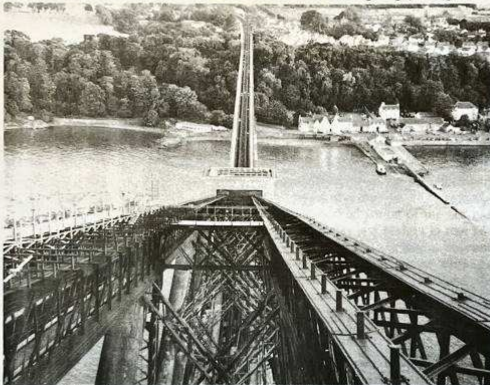
Figure 12 – Maintenance, September, 2000, with Rennie's Pier
