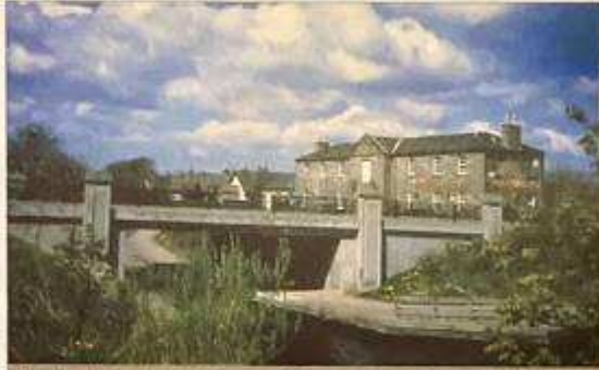
Fig. 12. Glasgow Road bridge, one of four constructed as part of the Glasgow Canal project in 1990 to provide adequate navigational headroom
