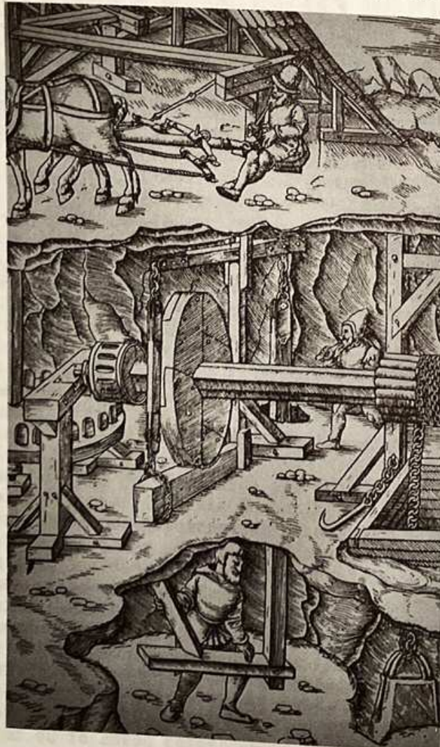
4 Horse-whim and machinery to mine shaft chain - Agricola 1556
