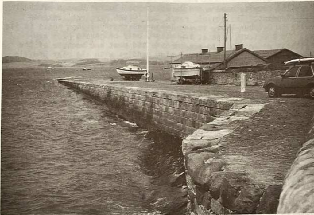
2 Longcraig Pier 1990 - Rennie, constructed 1816-17
