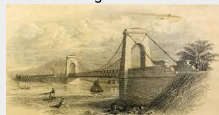
Left: Brown's ill-fated suspension bridge on the Darlington and Stockton Railway. See the article on the following page.
