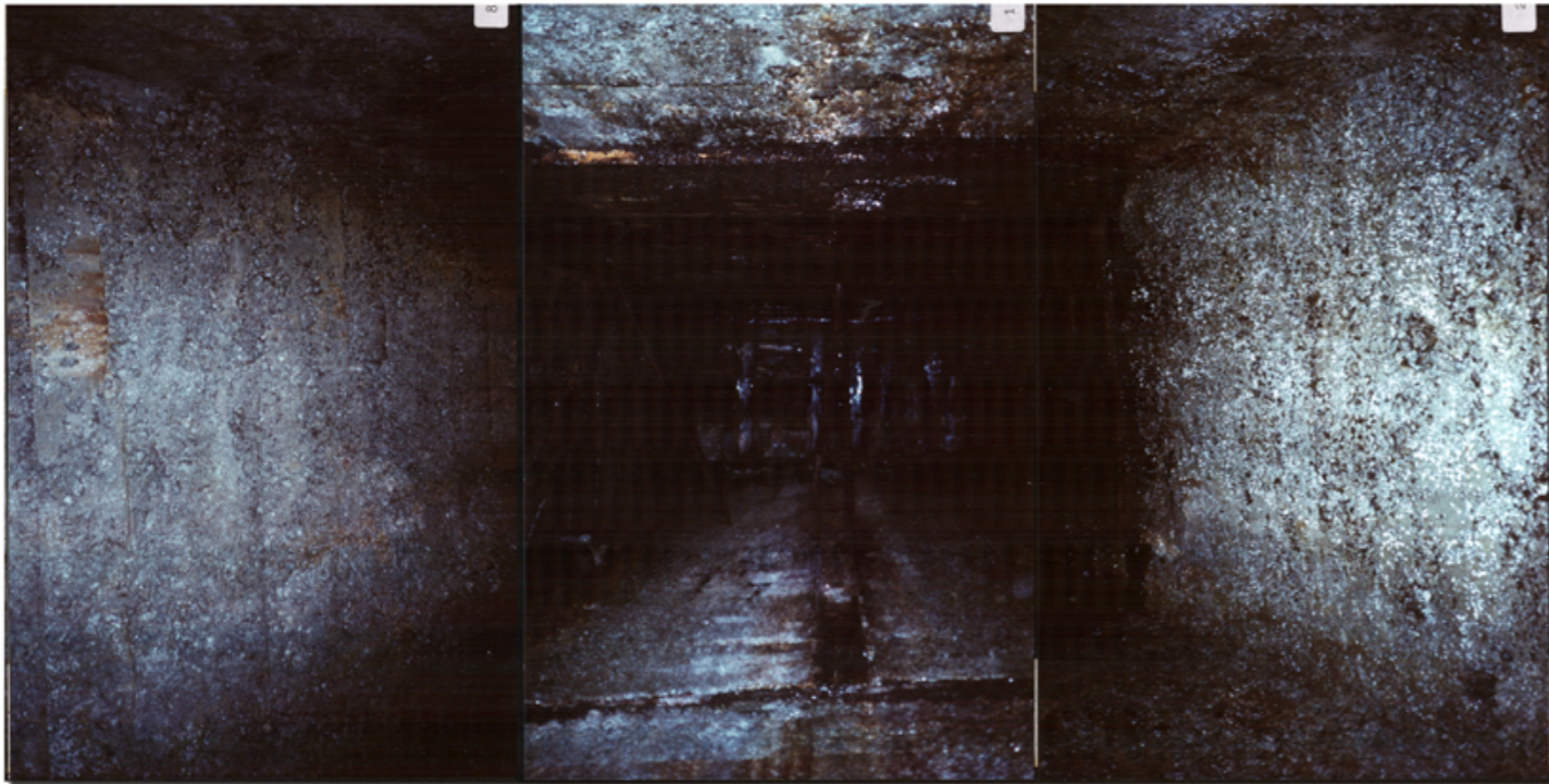
Glenfinnan Viaduct – Interior of Mallaig King Pier
