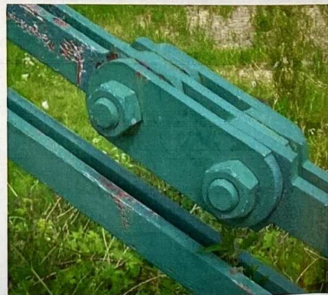
Fig. 4 Twin bar main chains with drilled eyes, and hexagonal nuts to cross bolts ©Redmore
