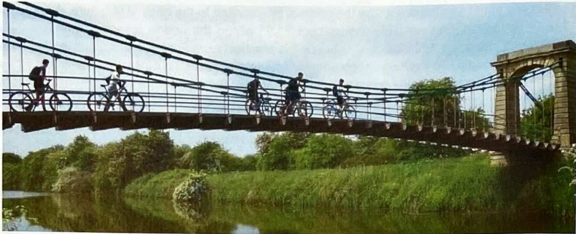
Fig. 10 Horkstow Bridge in recreational use in June 2021
