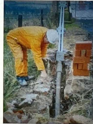
Fig. 6 Replacement of lower back chain ©Posford Duvivier
