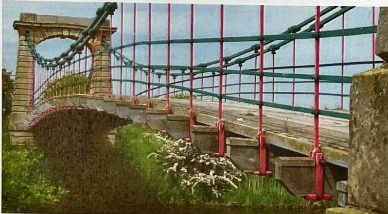
Fig. 5 Replacement deck in its original form utilising the 1836 ironwork © Redmore
