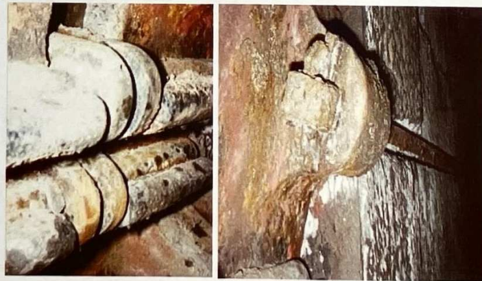
Figs 7-9 Cast iron chain anchor plate 920x1165x100mm in tunnel [Fig. 11] bearing on a substantial masonry wall [see Fig 9, from which the plate top in Fig. 7 was drawn, and Fig. 11] ©Redmore
