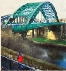
Wearmouth Bridge (1929) (engineer: Mott Hay & Anderson)
