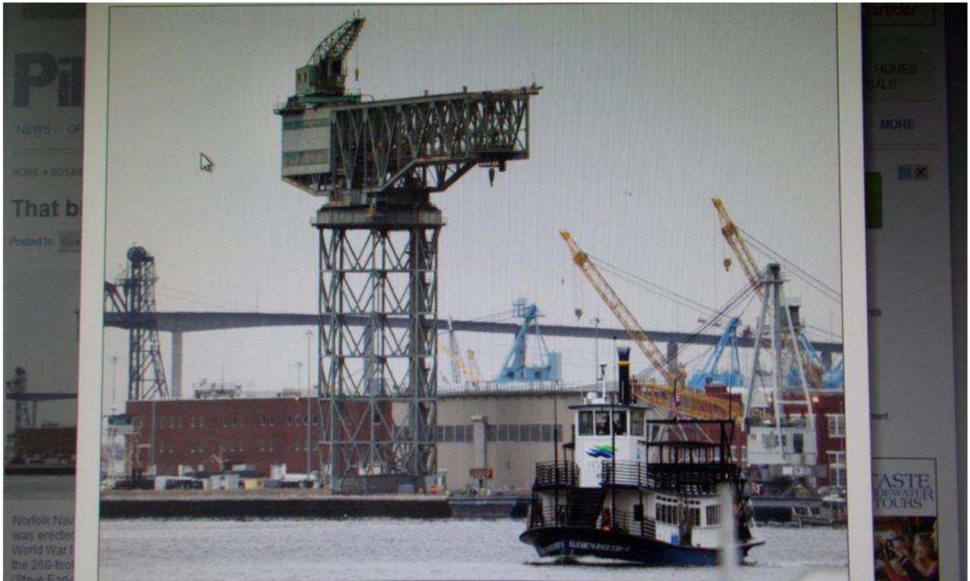
USA development. Giant Cantilever Crane, Portsmouth, Virginia, 300-ton, 1941 – now disused [www 28.6.13]
