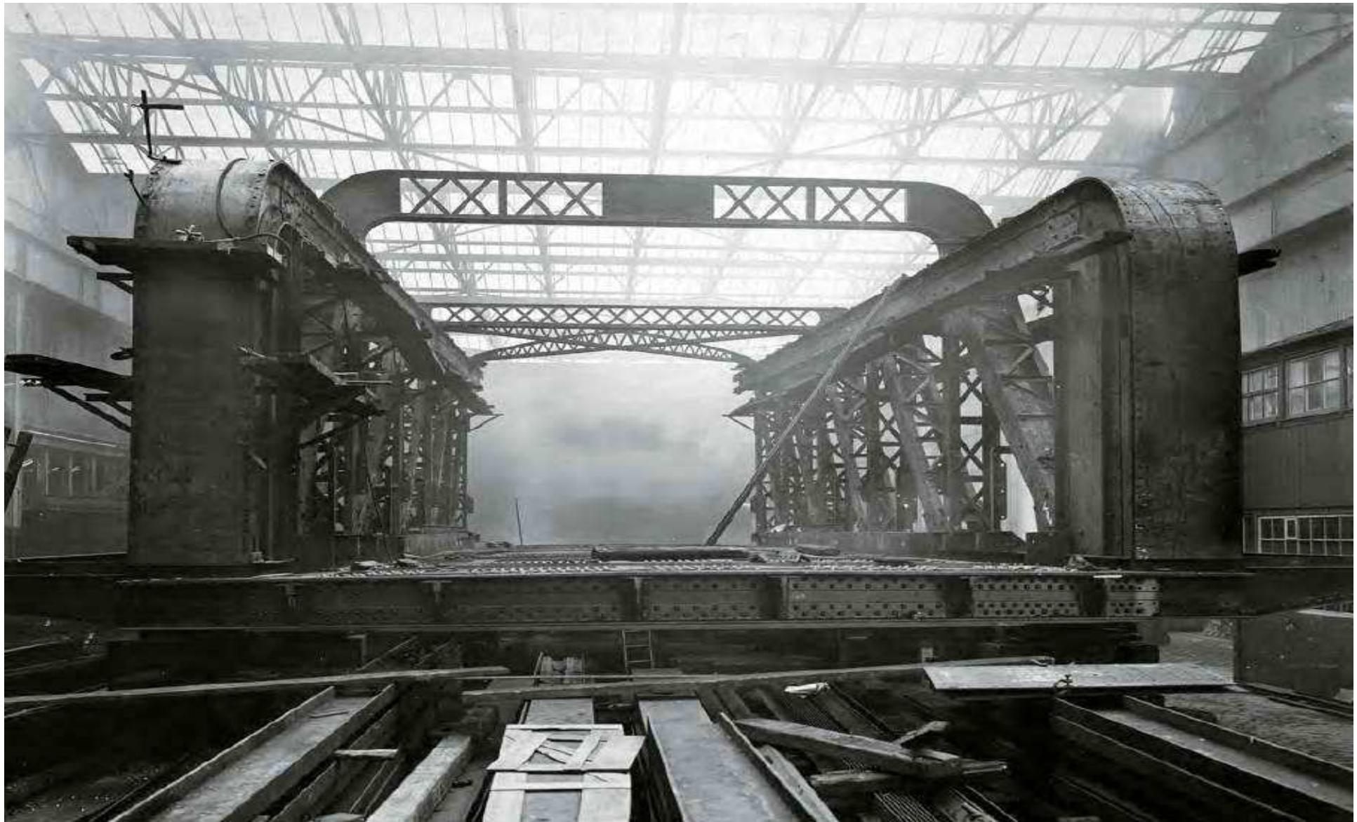
Albert Docks Swing Bridge – Dalmarnock Iron Works 1919 Many other swing bridges erected [RCAHMS 2000, pl. 85]
