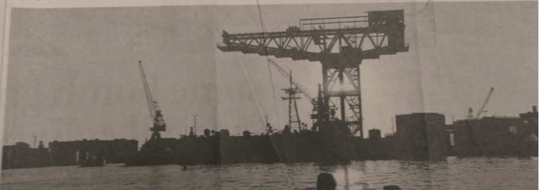
Giant Crane, Sydney, Australia, 1951 – 250-ton, disused - the penultimate Titan? [Belfast, 1958] [Sydney Morning Herald 29 March 2013]
