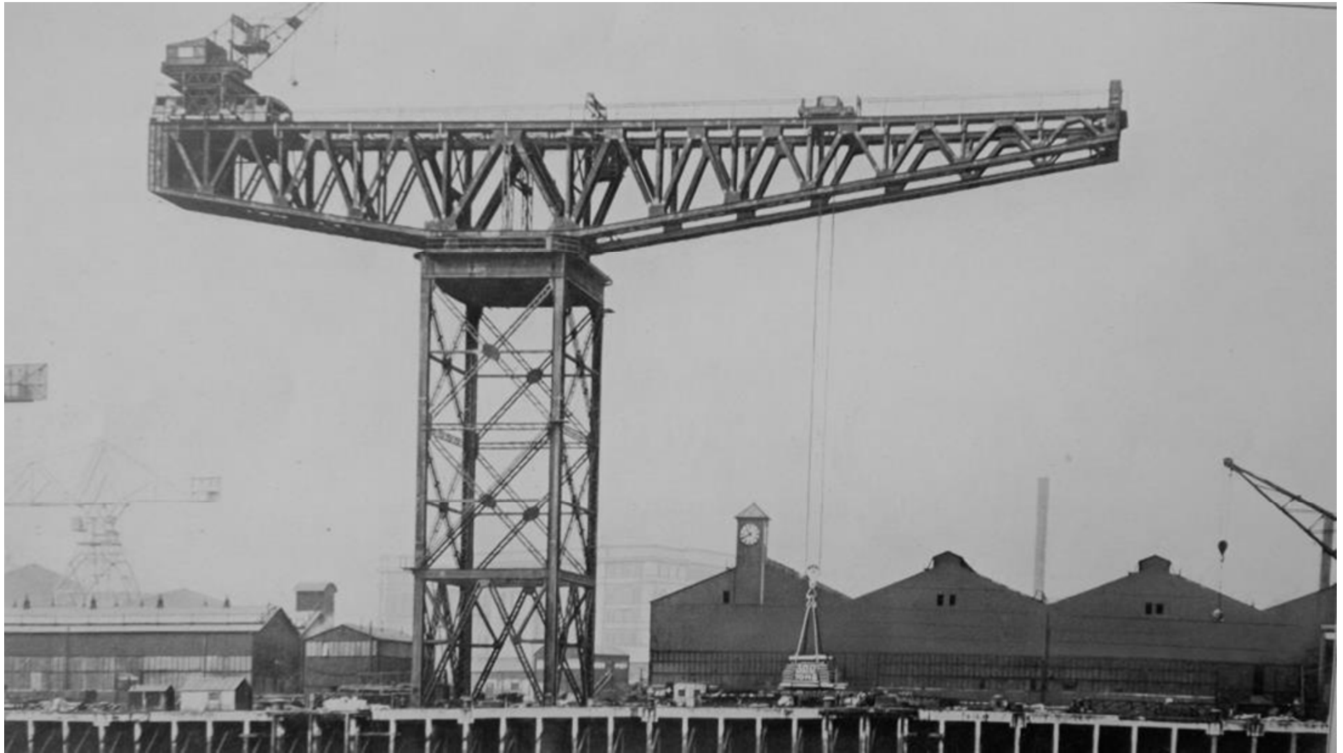
Walker Shipyard Crane, Newcastle-upon-Tyne under 300-ton test load in 1931 [Arrol Brochure – Hunter Archive]
