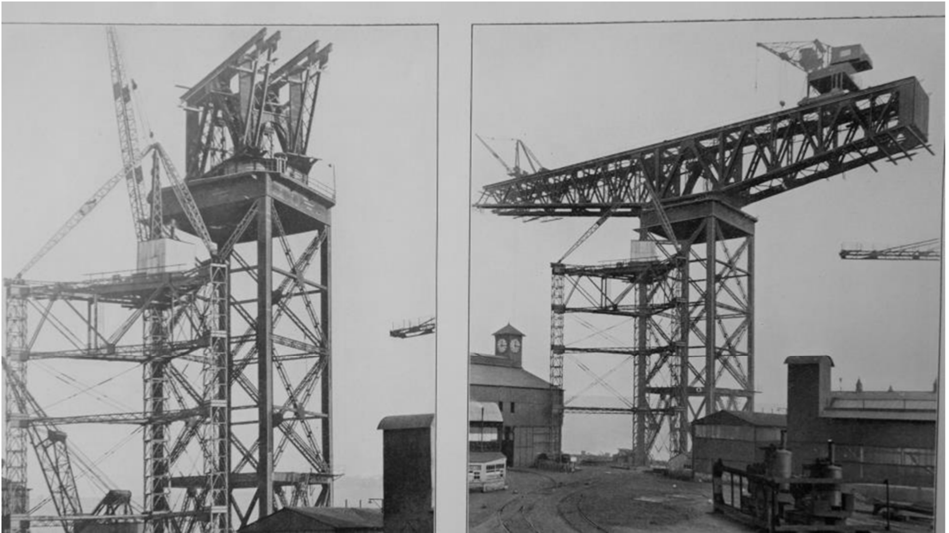
Walker Shipyard Crane 1931 – mode of erection by a derrick on a stand and balanced cantilever construction
