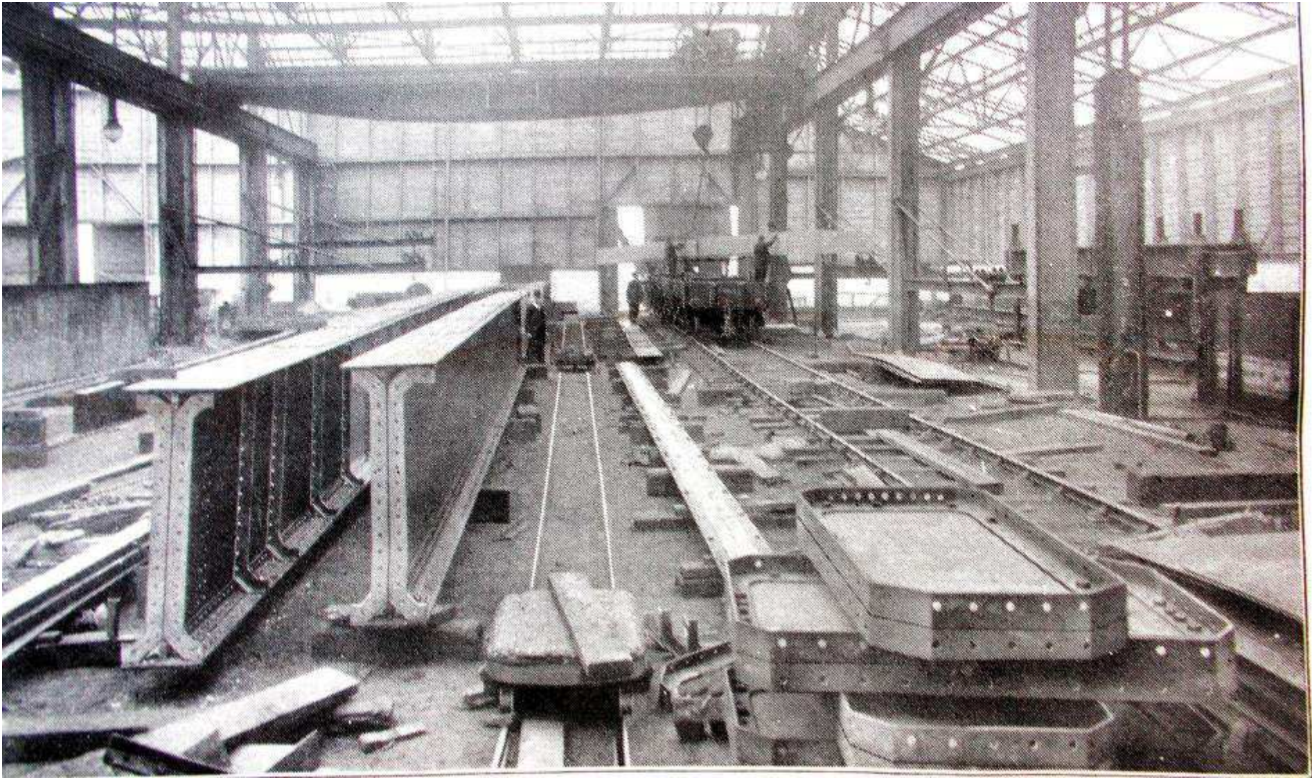
Arrol's Girder Fitting Shop, Dalmarnock Iron Works, Glasgow – loading arrangements in 1906 [Hunter 1906 pl. 18 – Hunter Archive]
