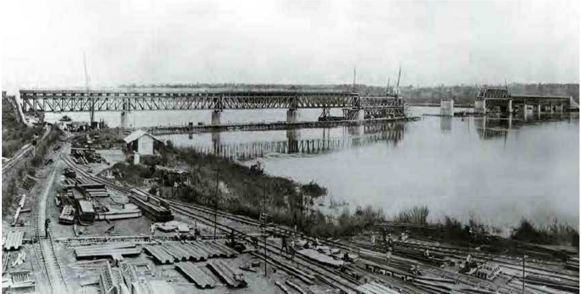
Benue Bridge [road/rail], Makurdi, Nigeria - 2584 ft long - nearing completion c.1930. Still in use, recently painted
