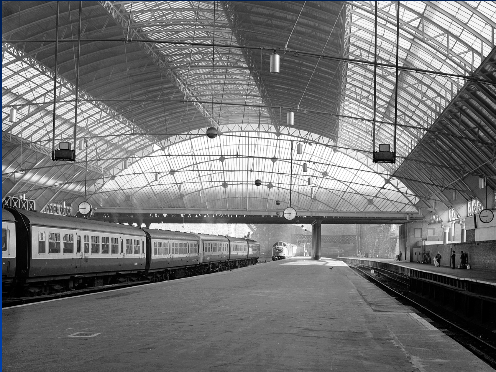
Queen's Street Station Roof, Glasgow 1879 (170 ft span)
