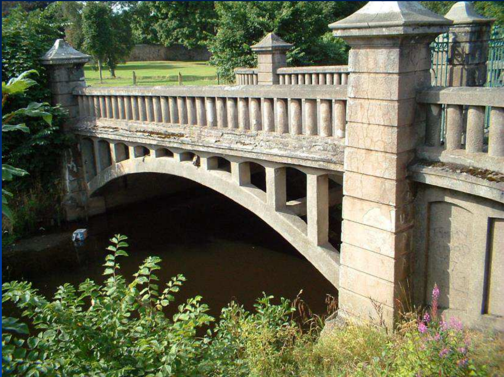
Saughton Park Bridge, Gorgie, Edinburgh 1907 (Mouchel 30 ft)
