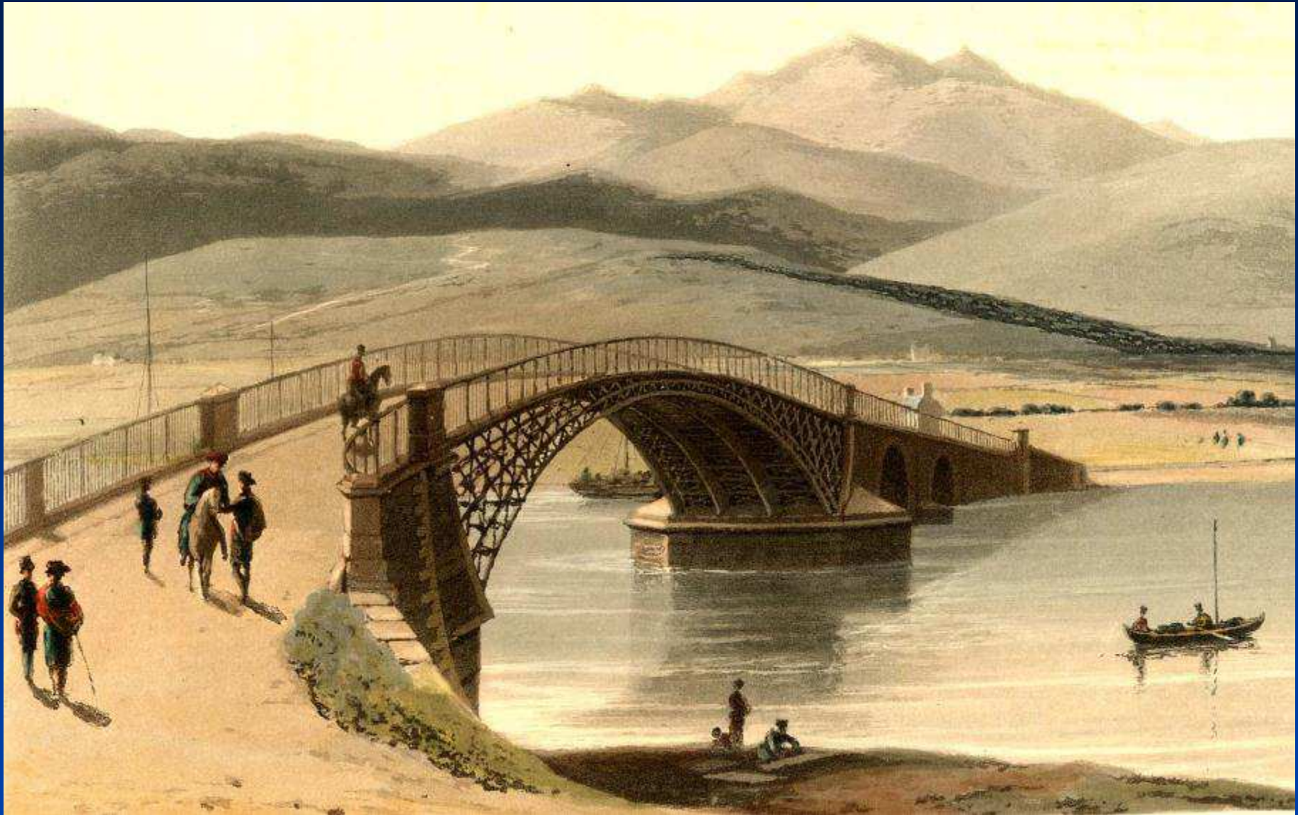
Bonar Bridge 1812 – Telford – First of a new innovative genre
