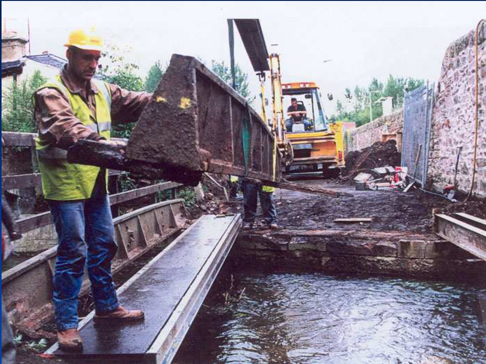
Edinburgh and Dalkeith Railway – Lifting Braid Burn Bridge (1831) in 2001
