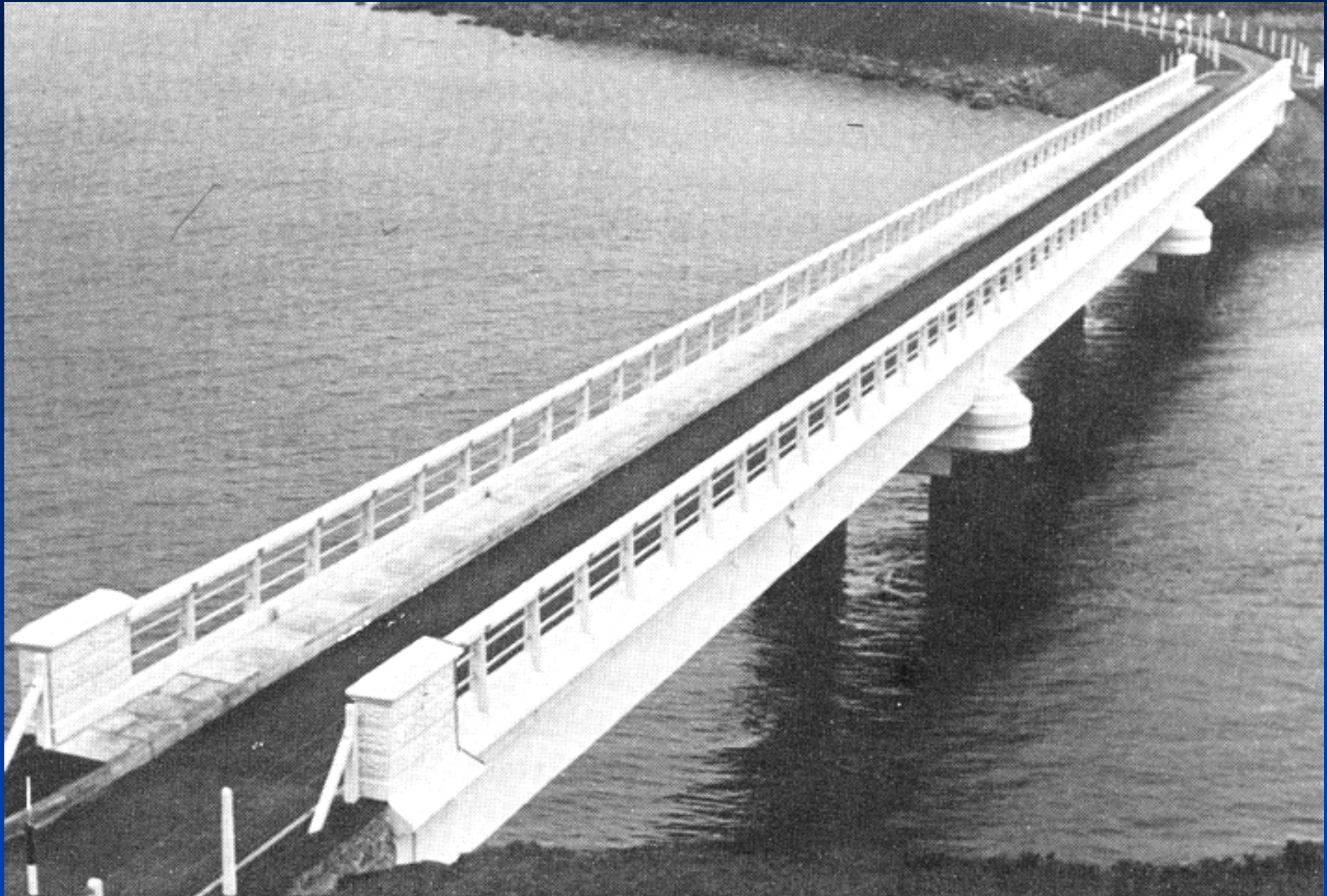
Bernera – Lewis Bridge 1953 – First pre-stressed example in UK
