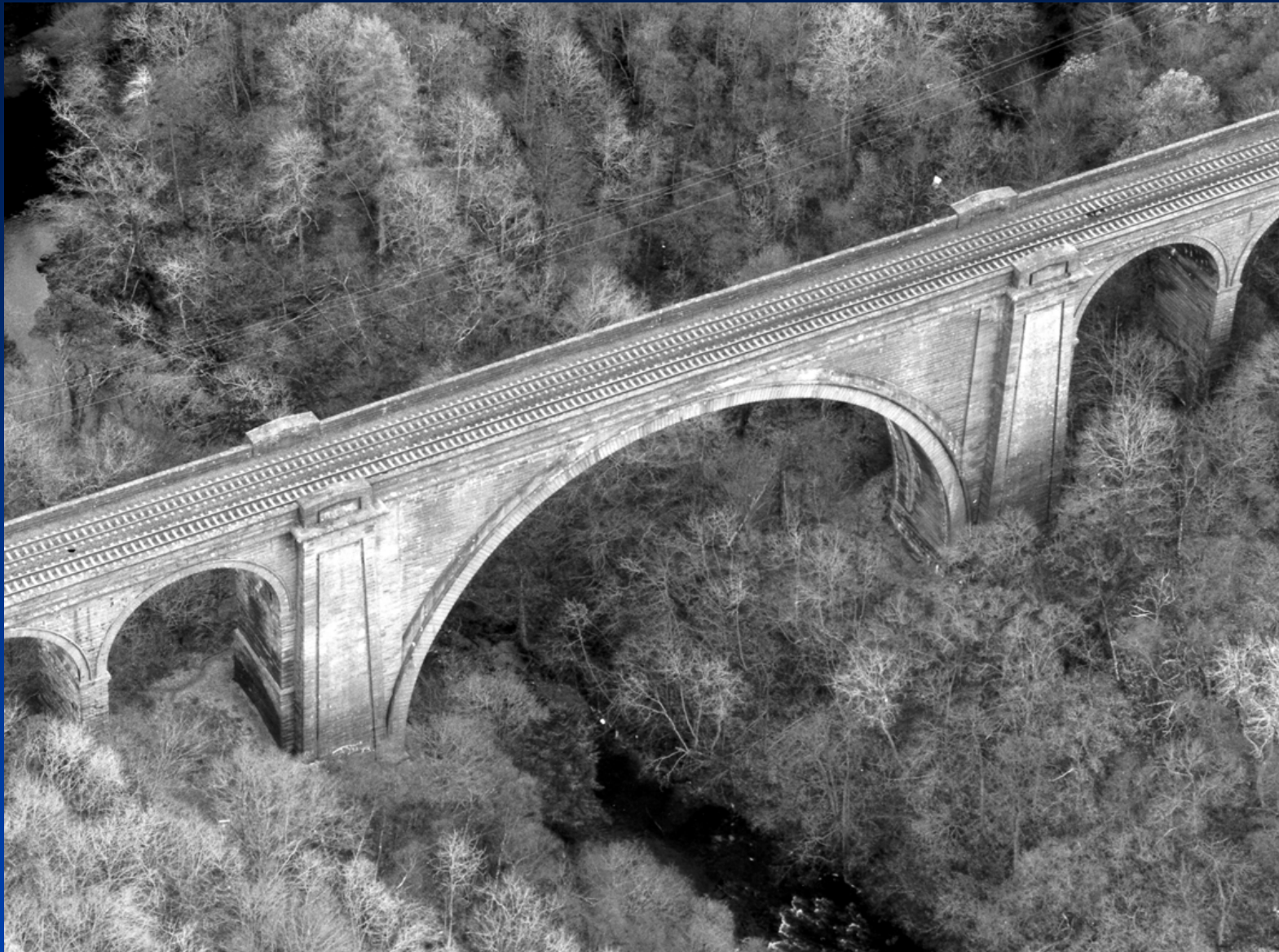
Ballochmyle Viaduct 1848 (181 ft span; 164 ft high)
