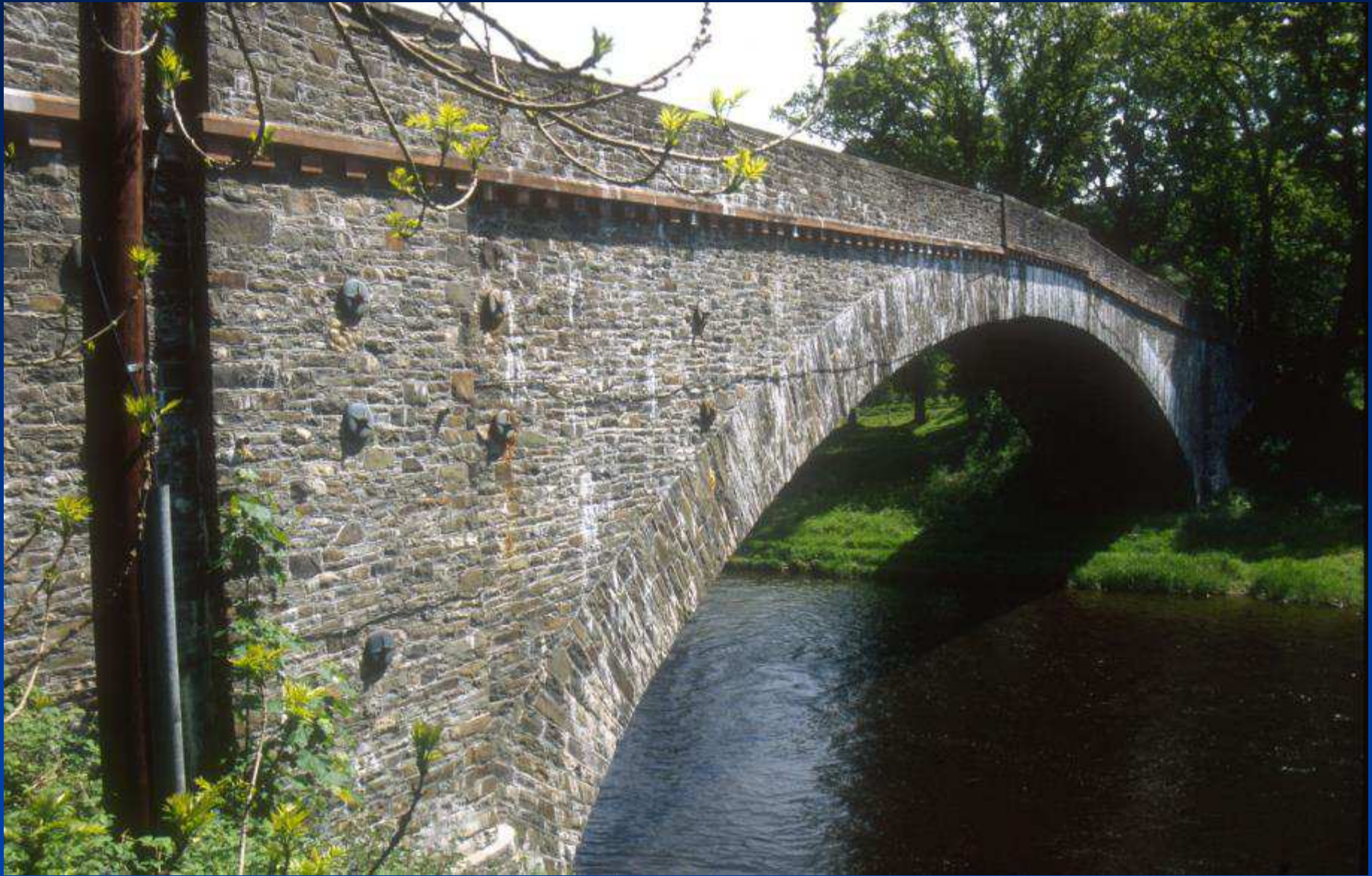
Ashiesteel Bridge 1848 (132 ft) (longest rubble masonry span in Scotland)
