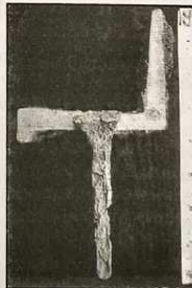
Fig 6. Whinstone block (above) and Glenbuck plate rail and spike c1810 found on site.
