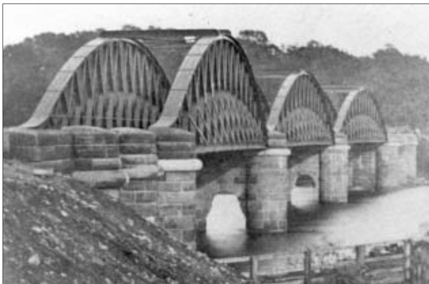
Loch Ken Viaduct
