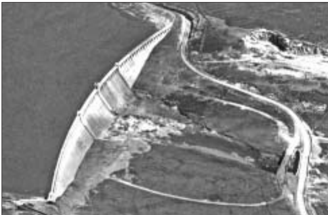
Altigraph Ltd, Scottish Power Generation Ltd
