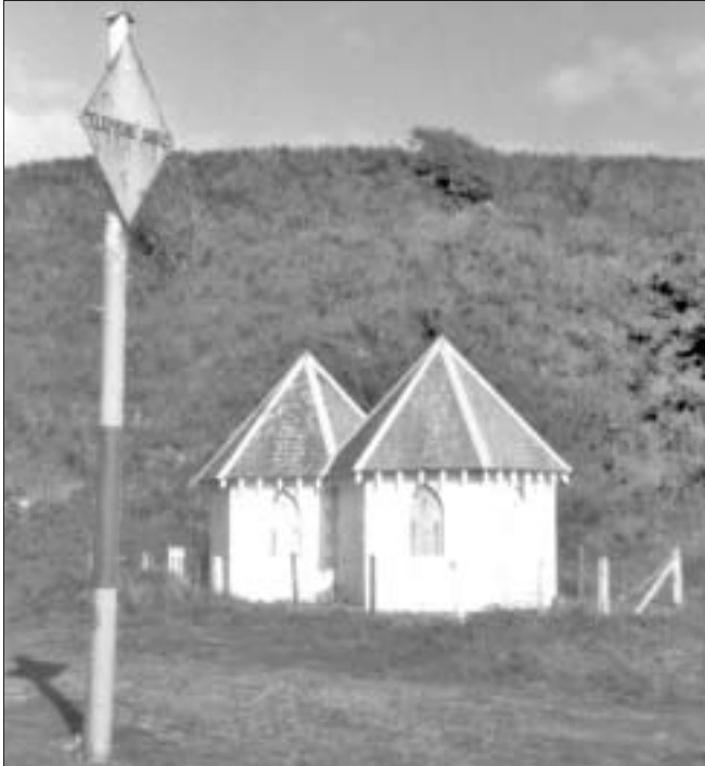
Laird's Bay cable house and marker
