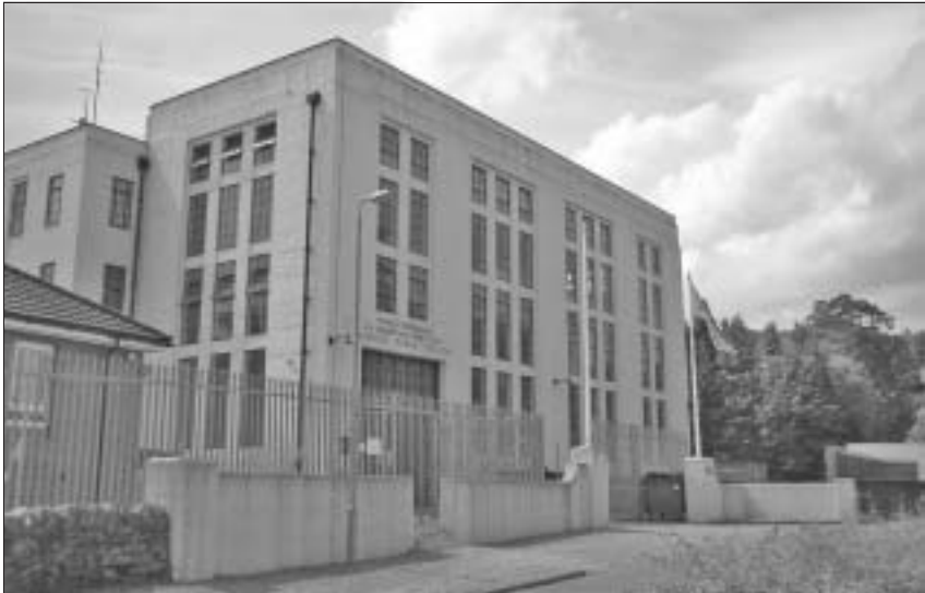
Glenlee Power Station
