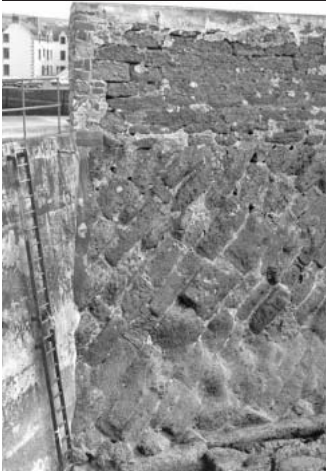
Eyemouth Harbour Pier – inclined masonry
