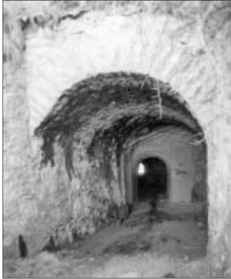
Cove Harbour Tunnel
