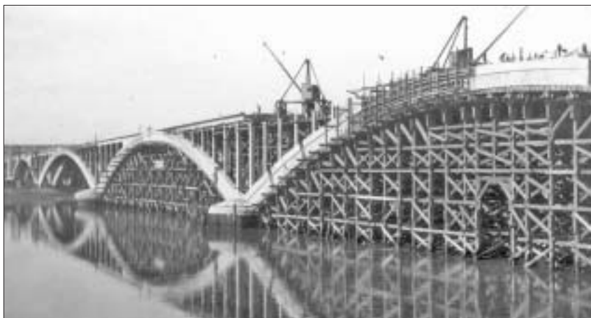
Royal Tweed Bridge under construction [postcard 1927]
