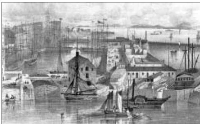
Leith Docks 1838 – entrance lock 1806 on left adjoining slips and dry dock [lithograph 1838]
