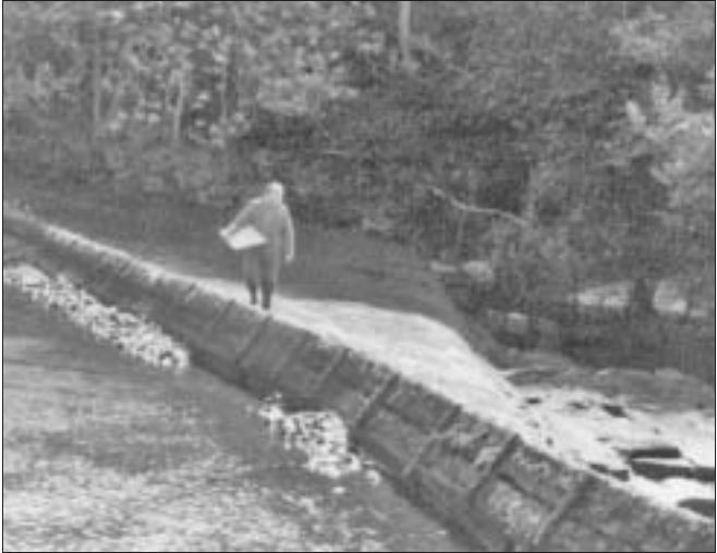
New Lanark Clyde Timber Dam [61]
