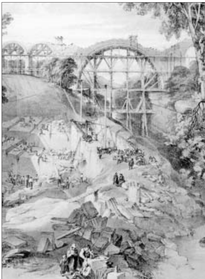
Ballochmyle Viaduct under construction [lithograph]
