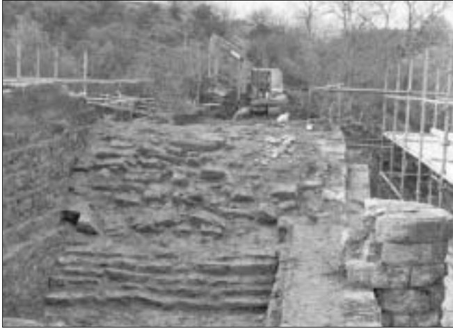
Laigh Milton Viaduct – internal construction revealed conservation
