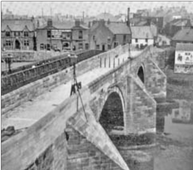
Ayr Auld Brig 1910 – preservation nearing completion. Note temporary timber bridge [8]
