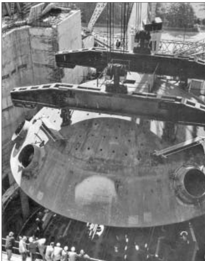
Hunterston 'A' Power Station – lowering pressure vessel top [22]
