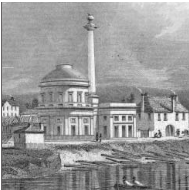
Perth Round House and pumping station 1832 [2]
