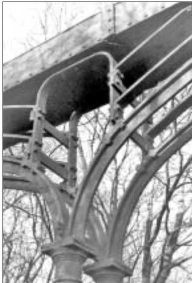
Slamannan Railway Aqueduct spandrel
