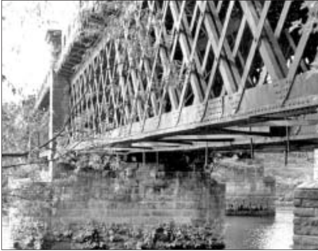
Downstream railway viaduct
