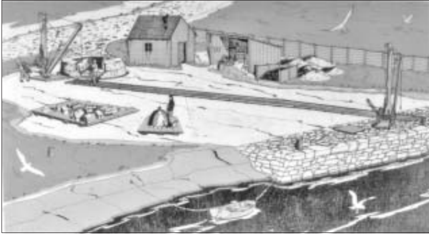
North Carr Rock Beacon workyard
