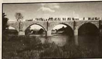
Laigh Milton Viaduct "after"
