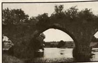
Laigh Milton Viaduct "before"
