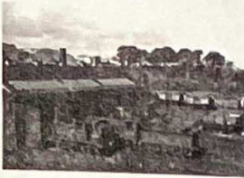
The locomotive depot at Polmont (date unknown), looking northwards. The Edinburgh & Glasgow Railway tracks ran this side of the shed. Photo: © Ben Brocksbank and licensed for reuse under this Creative Commons Licence
