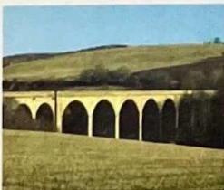
Roxburgh (Teviot) Viaduct was constructed as part of the Musselburgh branch of the North British Railway (1847). Unfortunately, part of it collapsed during the works, killing eight people.
