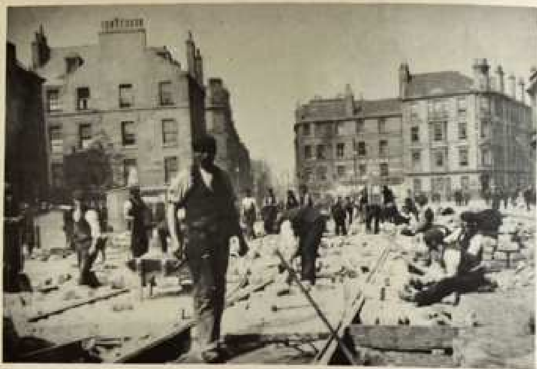
Sett Laying to Tram Rails at the foot of Leith Walk—c.1905 exhibit 57
