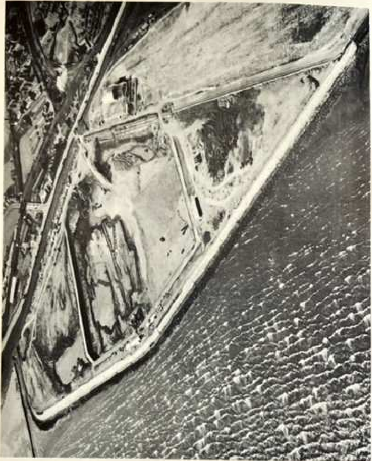
Sewage works under construction on reclaimed land
