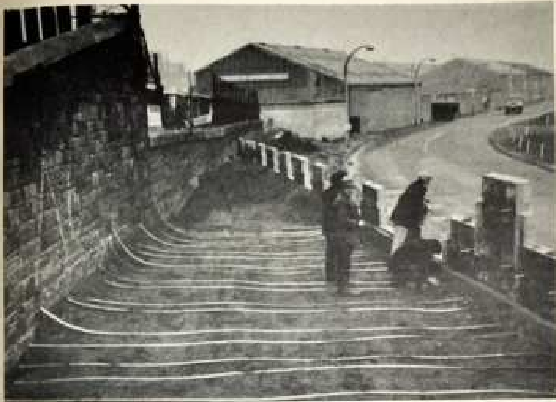
'Terre Armée' retaining wall under construction exhibit 95
