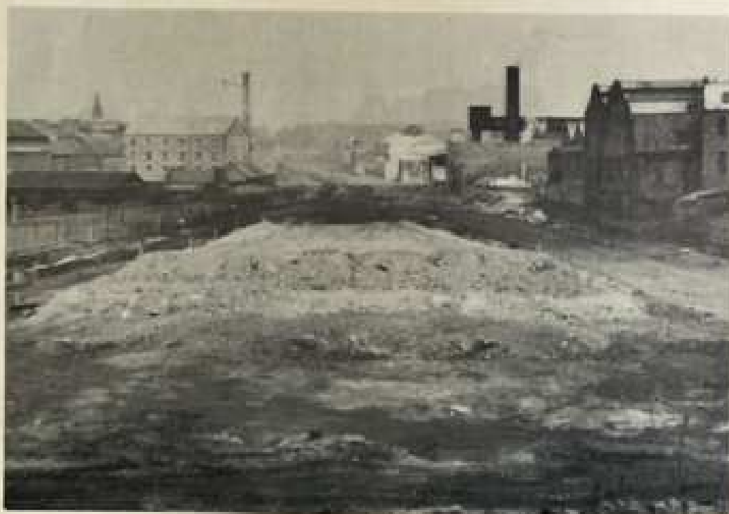
Edinburgh's first busway under construction exhibit 74-5
