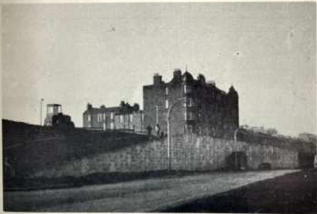
'Terre Armée' retaining wall nearing completion exhibit 97
