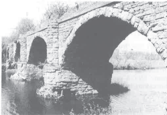
HEW 1469 West Gatehead Viaduct looking downstream
