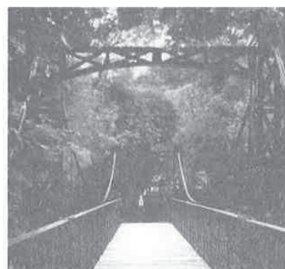
Crossford Footbridge over River Clyde near Carlisle made by P & R Fleming & Co., Glasgow, 1897
