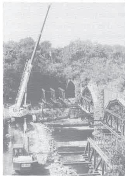
Laigh Milton Viaduct state of work 3 August 1995 looking west
