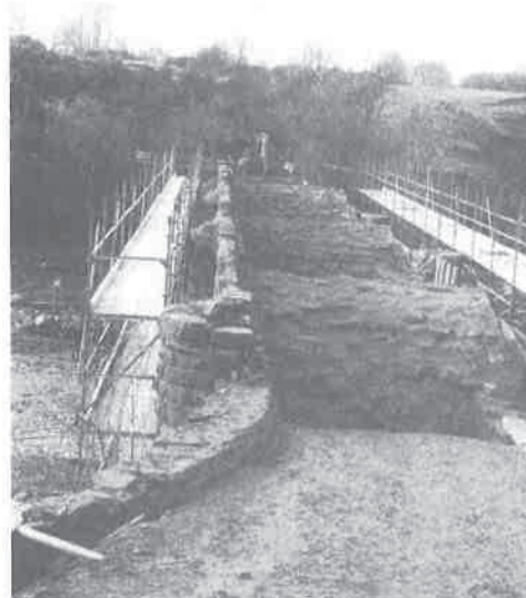
Laigh Milton Viaduct, 14 November 1995
